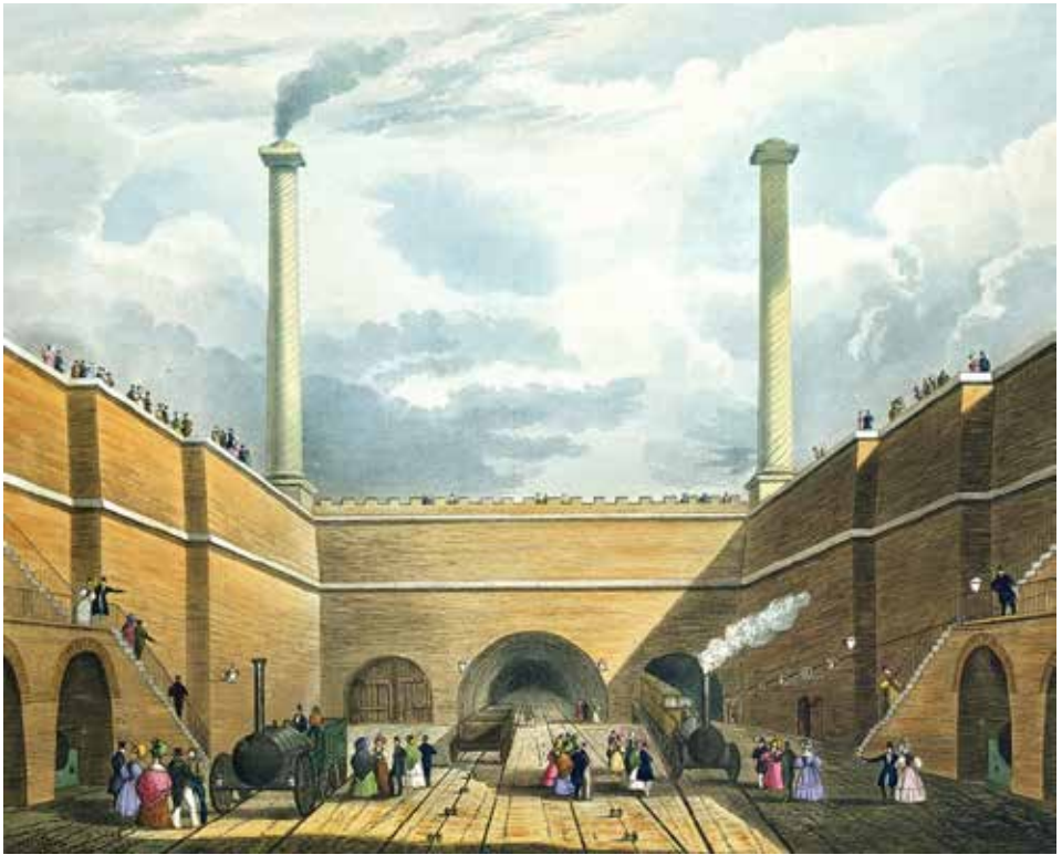
Edge Hill Station 1830. The centre tunnel was to the docks and the right hand tunnel served the terminus at Crown Street. Both tunnels were cable operated.
