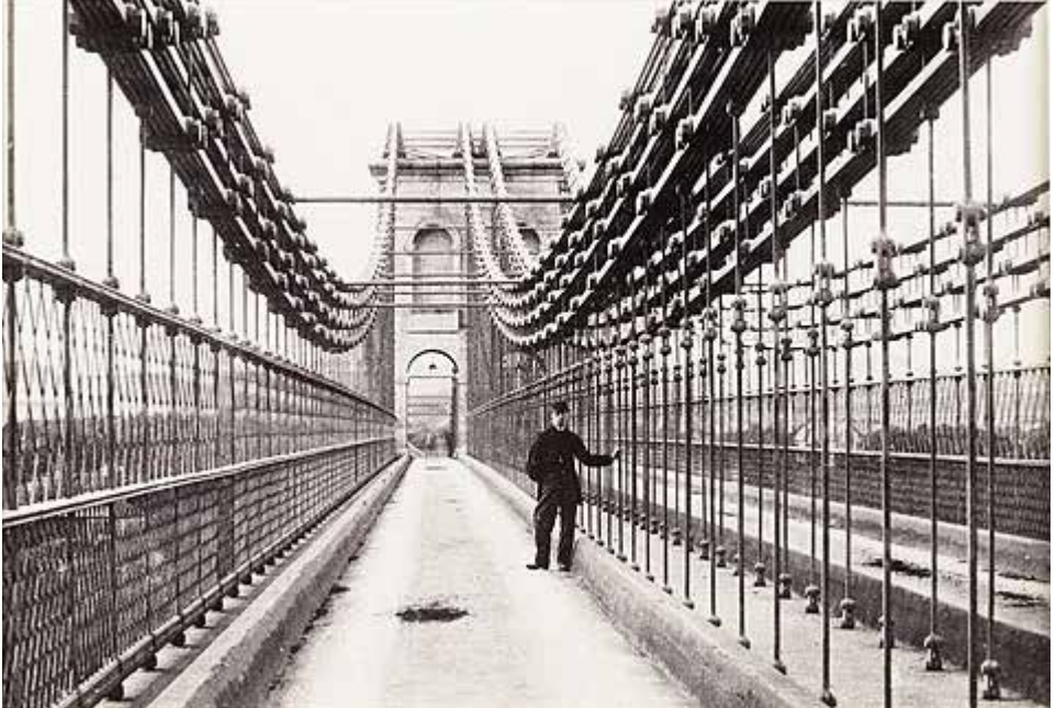
Menai Bridge showing original chain cables with wrought iron links. (Authors collection)
