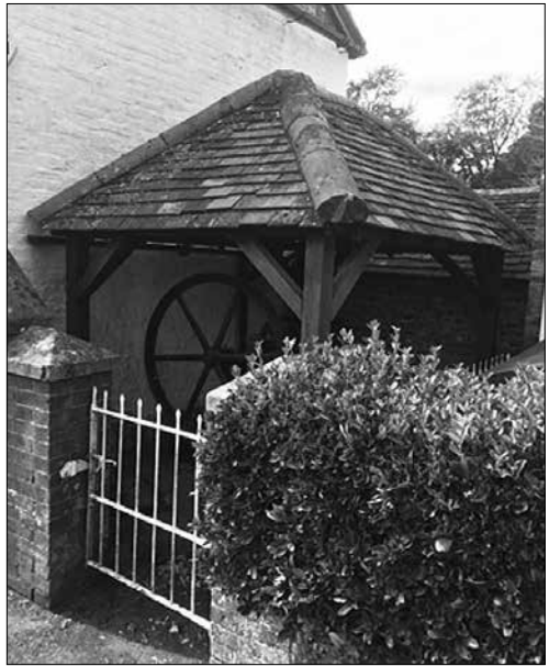
fig. 1 : The Findon Pump and Well House D. Dunkin
