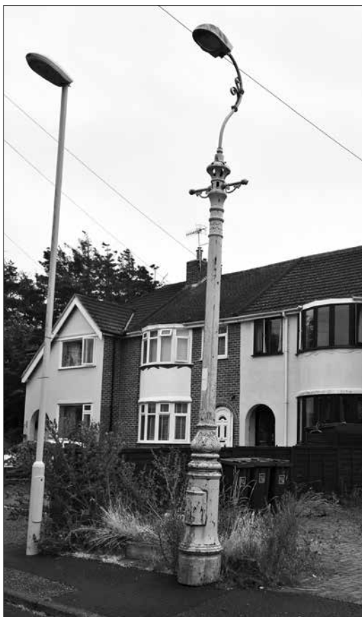
Example in Worthing, with a redundant lamp fitting. More often seen without a lamp (Martin Snow)
