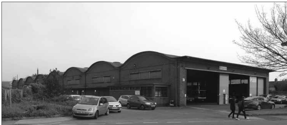
Fig 1 Chichester Bus Garage seen from Basin Road, the subject of the most recent SIAS listing attempt. (Alan Green)
