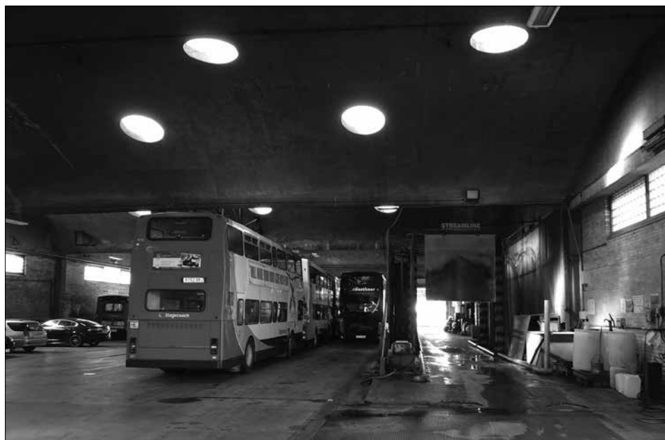
Fig 2 The interior of the garage on the occasion of the SIAS visit in 2016 which shows the unobstructed operating floor afforded by the clear-span roof. (Malcolm Dawes)
