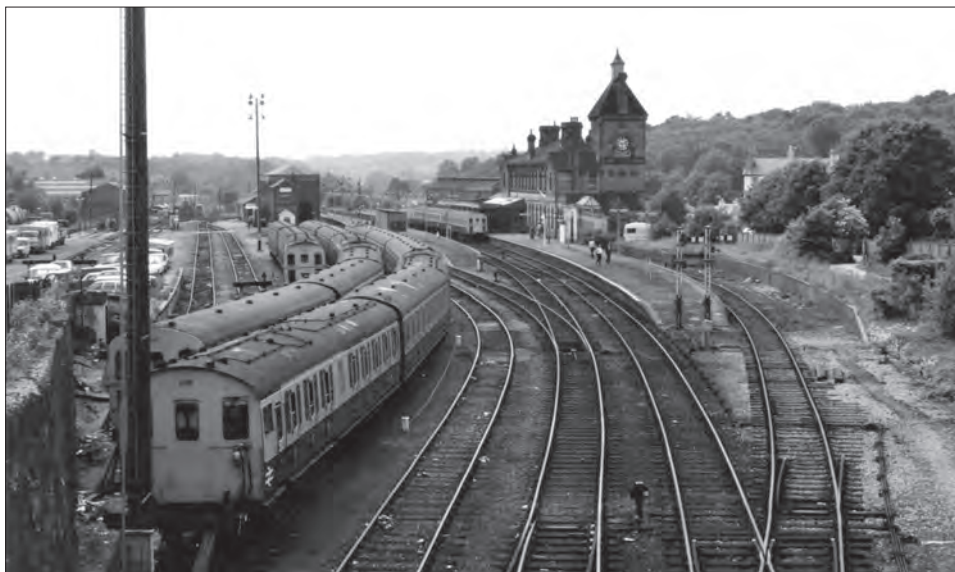
The view of Tunbridge Wells West from Montacute Road bridge in June 1985 just weeks before closure. By this time the island platform buildings and canopies had already been demolished and the canopy on the main station building shortened. The sidings are being used for berthing several 3H and 3D DEMUs. From this viewpoint today only the top of the clock tower is visible above the redevelopment that has taken place on this vast site. (Alan Green)
