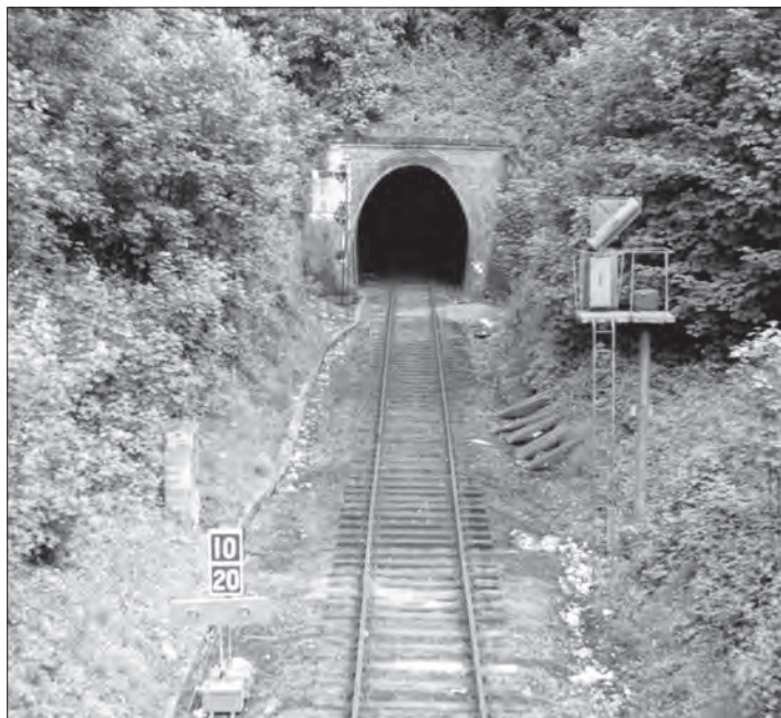
Grove (Frant Road) tunnel viewed from Montacute Road bridge in the early 1980s. The cutting is now heavily forested making this view now impossible. (Alan Green)
