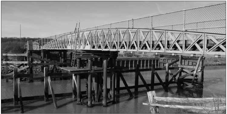
Fig 2. Southease Swing Bridge across the River Ouse, seen in 2009 when it was under threat of demolition and replacement by the Environment Agency. It was subsequently listed Grade II and saved. (Author)
