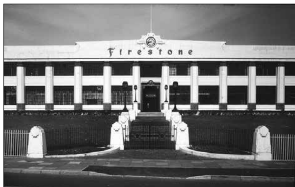
Fig 1 The former Firestone factory in Brentford, controversially demolished in 1980 just before becoming listed. This outrage demonstrated the Importance of Being Listed. ( 20th Century Society)
