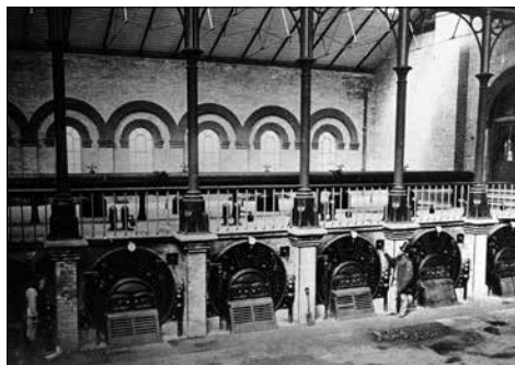
Crossness original 12 Cornish boilers
