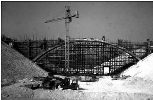
Adur Flyover - Mill Hill Bridge under construction
