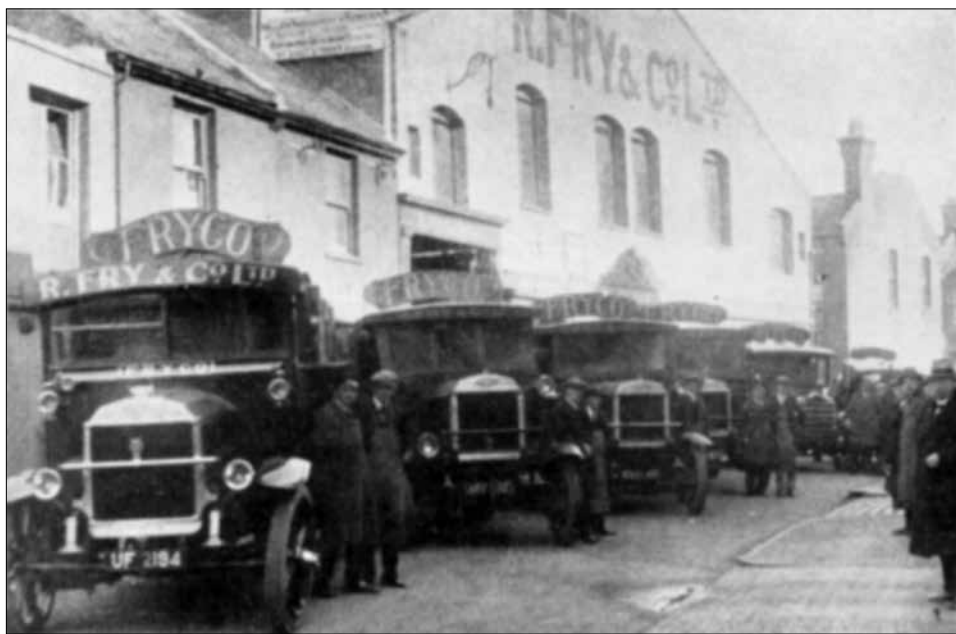
The Park Crescent Place frontage of the former Gaiety Theatre after conversion for Fryco Ltd
