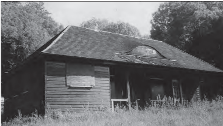
The tea house at Fairmile Bottom on the A29 N.W. of Arundel. Now happily moved and restored to its original use at nearby Amberley Museum
