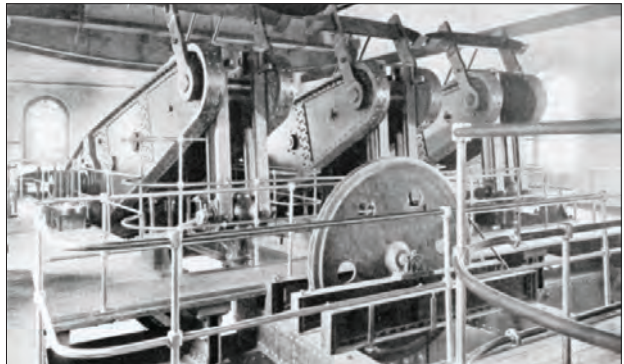
Severn Tunnel beam engines
