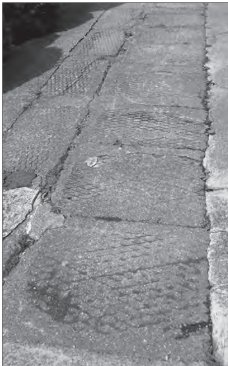
The Path at King Charles Cottage, showing the metal reinforcement (John Blackwell)
