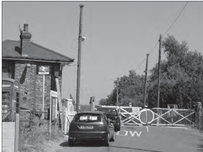
The Warnham level crossing gates from the west, after re-signalling in 2005 led to their permanent closure. Note the signal box leaning on a wooden crutch. Both are gone now, see back cover for a recent view.
