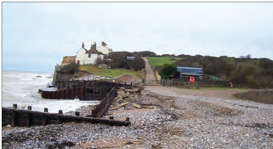
The former coastguard cottages at Cuckmere Haven with the cable hut at the right. This view from January 2014 shows the encroachment of the sea: refer to article inside.
