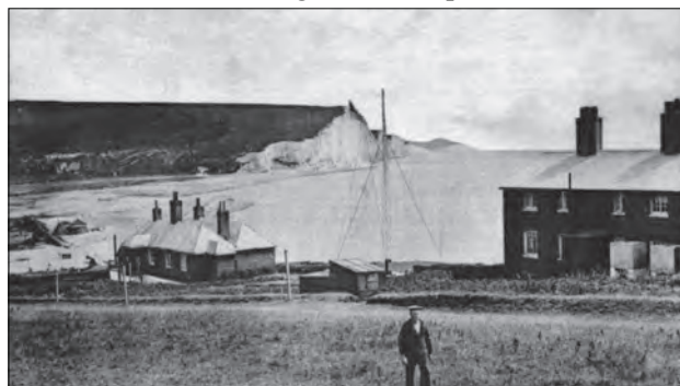
This old scene shows the properties when coated in black bitumen. The water tanks are shown by the doors.
