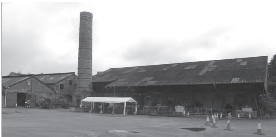
The northern aspect of the preserved buildings shewing, to the right of the chimney, the kiln block.
