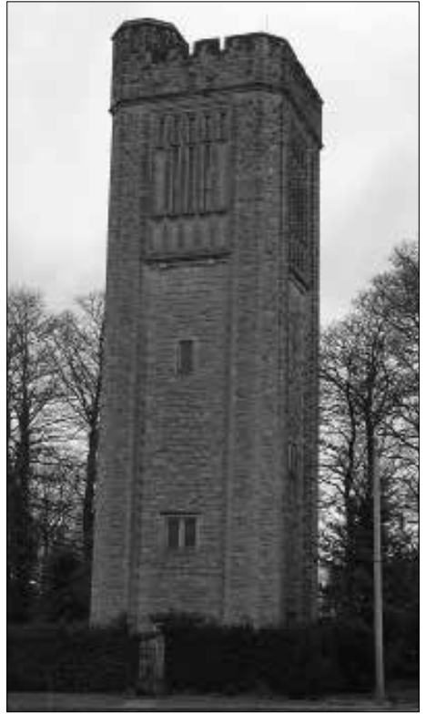
East Grinstead, Sackville Tower, Listed II now in a carpark and in domestic use.
