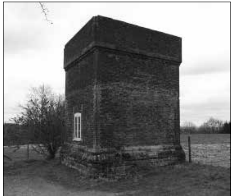
Turners Hill, overlooking the Weald close beside the B2110.
