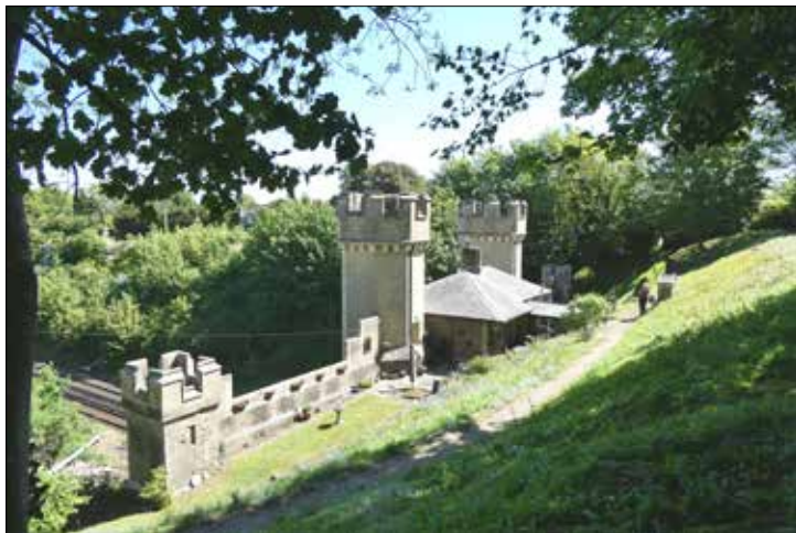
The rear of the portal shewing Tunnel House – note the rear outshot which most likely predates the main body of the house. On our last visit this part of the grounds was overgrown and inaccessible: much has been achieved since then to create this terraced garden. (Author)
