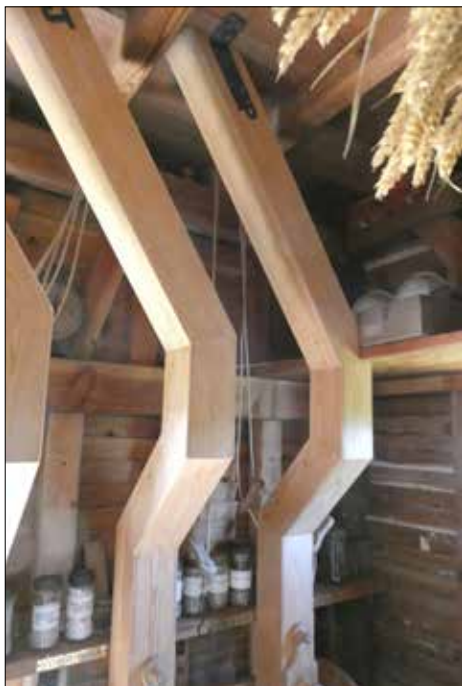
Some of the new timber spouts seen on the spout floor. The craftsmanship in the joinery is superb, - indeed it looks more like the work of an organ builder but is, in fact, the handiwork of one of the volunteers. (Author)
