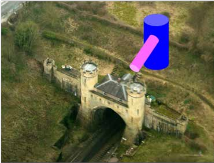
A CGI produced by David Porter shewing the position of the adit and the blocked-off construction shaft. This aerial view also shews how much clearance work has been done to create the terraced garden. © David Porter.
