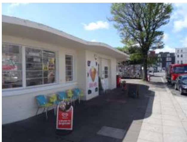
Fig. 2 The west side of the shelter today. The breakfront section housed the original open entrance to the shelter but has now been blocked up. Note how the overhanging roof stylishly sweeps out to accommodate the breakfront. ( Author )
