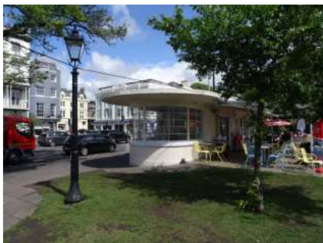
Fig. 3 The south end of the shelter shewing the apsidal end and the curved Crittall windows. The patio of the café now occupies the area that was once the ventilation block for the public lavatories. (Author)
