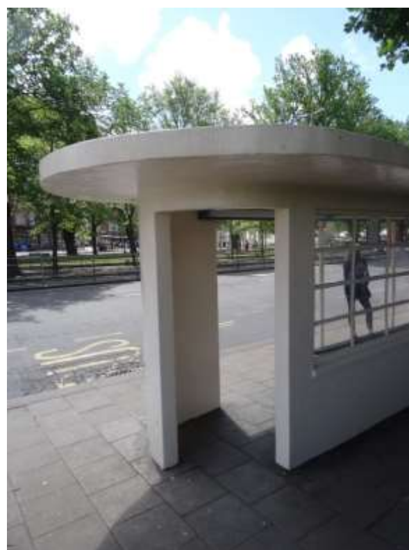
Fig. 6 The north end of the bus shelter shewing the very wide overhang of the reinforced concrete roof, and the entrance which takes up half of the apse. (Author)
