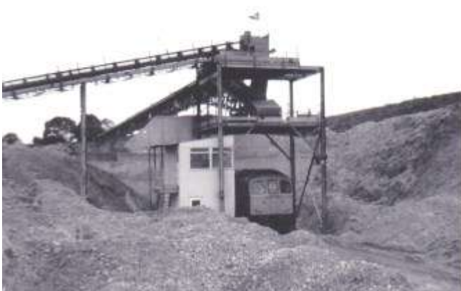
Fig. 20 Loading gravel at Lavant in June 1973. There is no landmark in this picture to locate this rather desolate quarrying scene, but it is in the vast new gravel pit south of Snakes Lane. The 'Crompton' is sitting below the loading plant and will slowly draw its wagons forward for charging. (Author)
