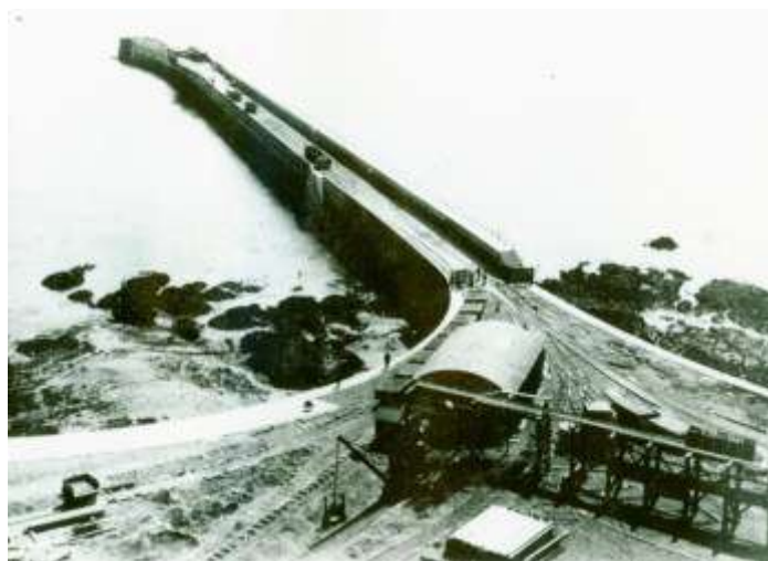
Fig. 12 The part-finished breakwater about the time of the 1883 'crisis'
