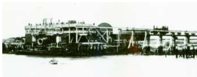
Fig. 6 Cement mixer and hopper barge, East Quay
