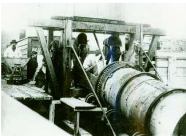
Fig. 10 Mobile concrete mixer on the breakwater (see also fig. 2)
