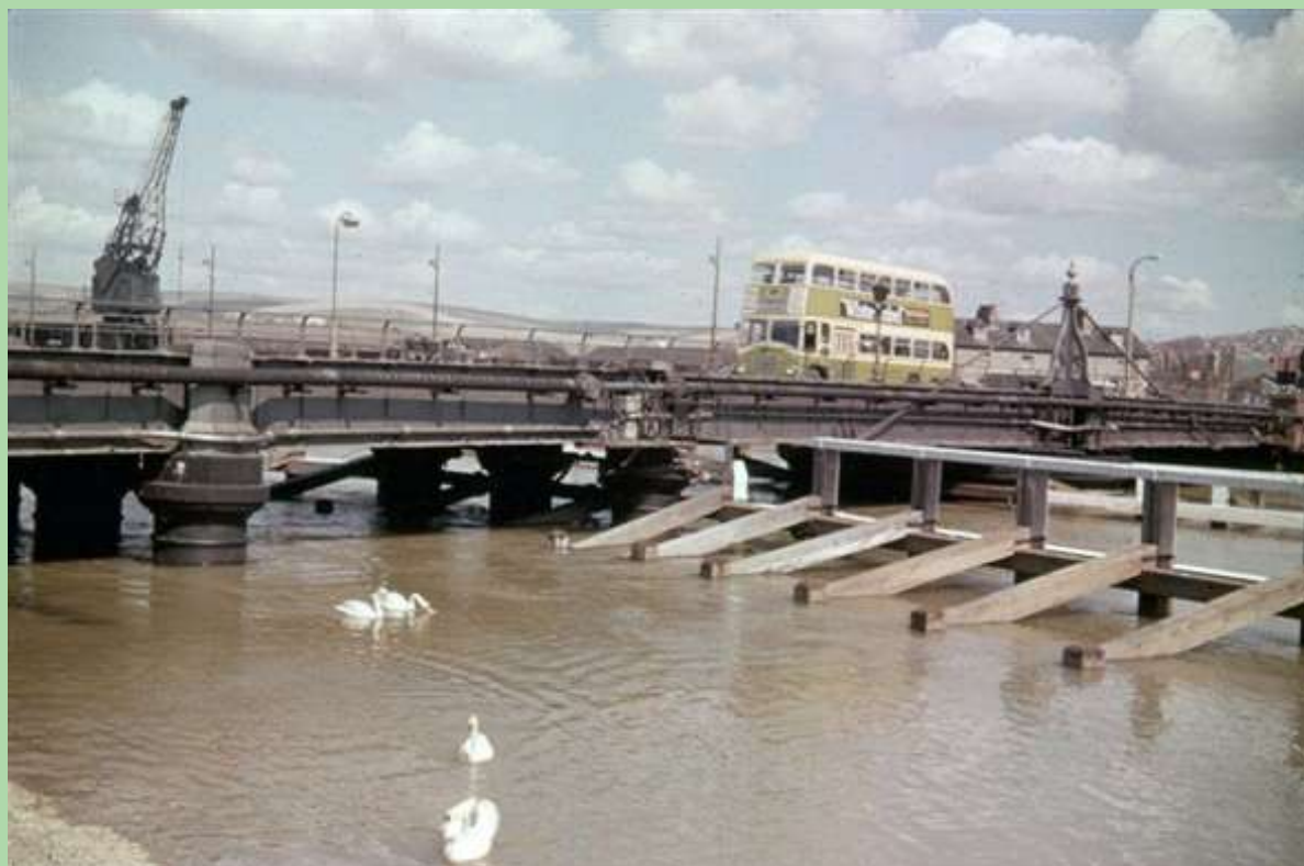
Newhaven Swing Bridge, looking east ( photo: John Hoar )
