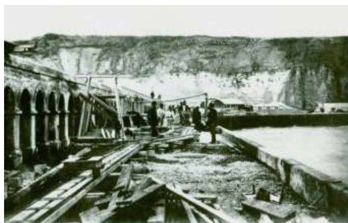
Fig. 3 Trip hazards abound – health and safety was clearly not a priority
