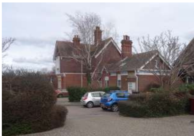
Fig. 23 The frontage of Lavant Station today. Comparison with Fig. 8 reveals the wholesale alterations carried out on its conversion to apartments, but the porch had been removed back in the 1930s (Author)
