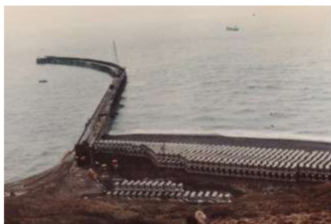
Fig. 14 'Bonios' stored west of the breakwater. Note the crane used to put them into position.
