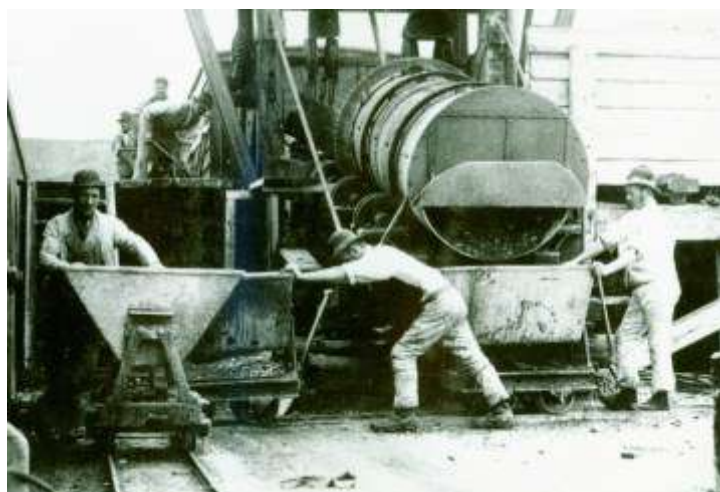
Fig. 2 Men working on the concrete mixer located on the breakwater
