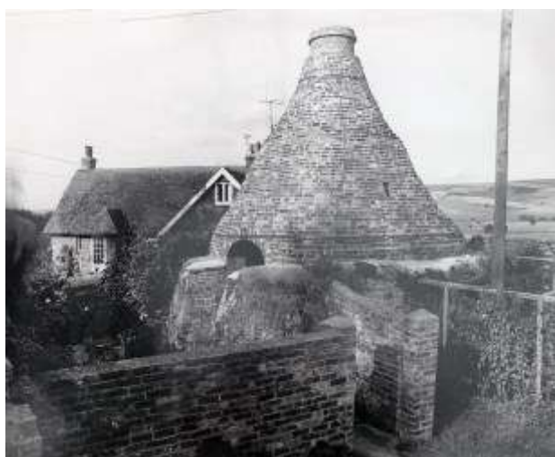
Fig. 9 Piddinghoe kiln after restoration (photo: John Upton)
