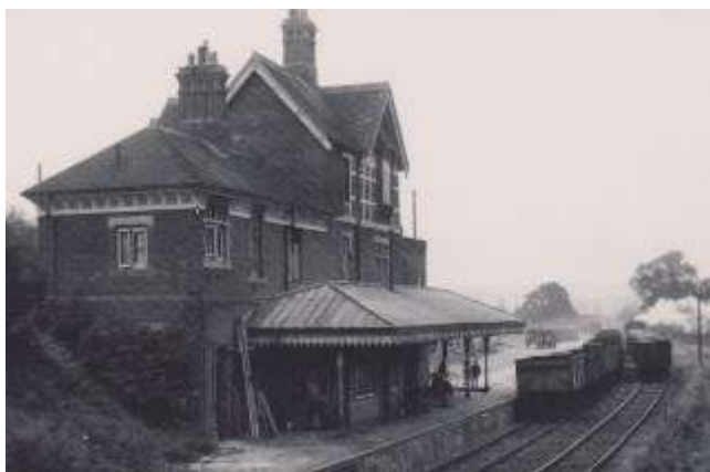
Fig. 18 A sugar beet train being shunted at Lavant by an unidentified loco in 1955. Mineral wagons are seen parked against the platform. ( S C Nash)
