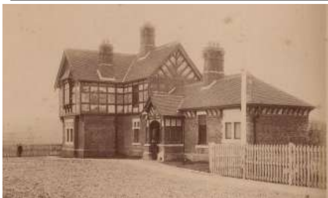
Fig. 8 The frontage of Lavant station from the same album. Although the station building has survived this view is unrecognisable today. (WSRO)
