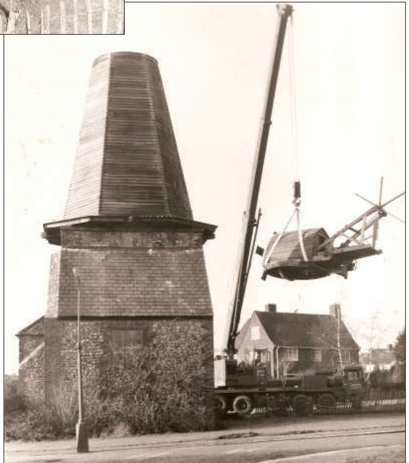
Fig. 8. Restored cap being replaced in 1983 ( Author's collection )
