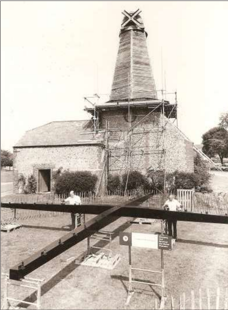
Fig. 7. Painting new steel stocks, 25 Aug 1980 ( Brighton & Hove Gazette )
