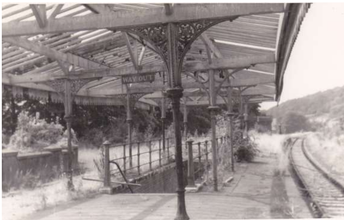
Fig 17. The sorry scene of dereliction at Singleton after freight services had ceased and the demolition men were awaited. This is the down island platform looking towards Chichester with the water tower visible in the middle distance. Most of the glass has gone from the canopy and several of the valance boards have dropped out giving a gap-toothed appearance. Hardly fit for royalty now. (Author's collection)
