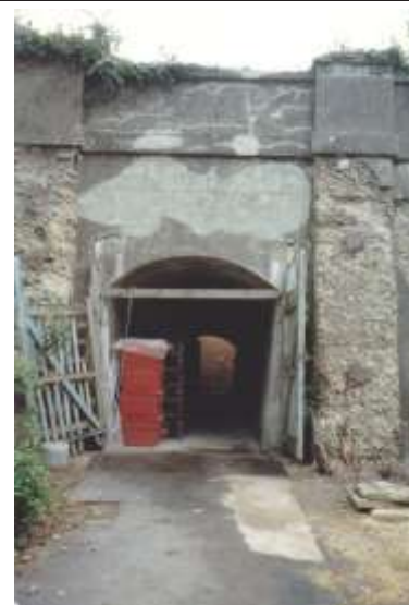
Fig 11. The entrance to the subway seen in 1981. Most of the render has fallen off the retaining wall revealing the rough mass concrete behind it. (Author)
