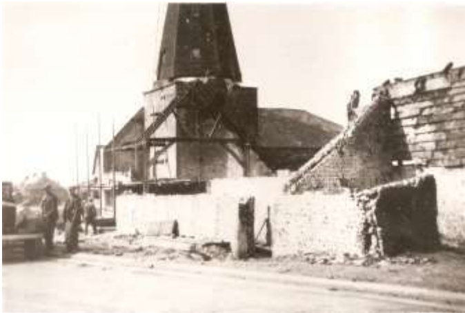
Fig. 4. Demolition of the old north barn in 1938, clearly showing tall flint & brick tower predating mill by 75 years ( Author's collection )
