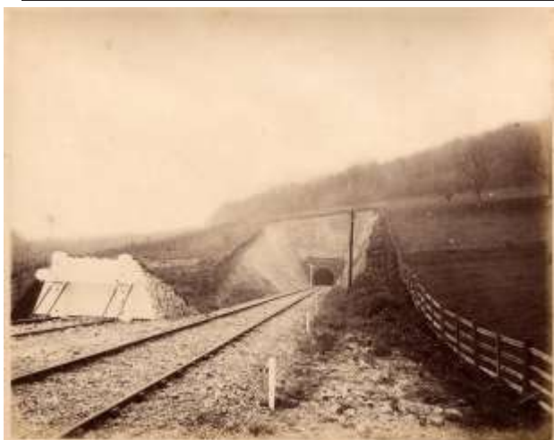
Fig 5. The country-end approach to Singleton taken from Banister's album. To the left is the buffer stop to the down carriage siding, and in the background is the portal of West Dean tunnel whence the line rises at 1 in 75. The picture, taken on completion of the line in 1881, shews how raw the earthworks appeared when new.
