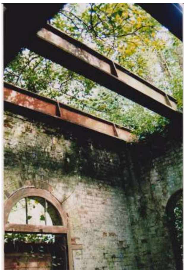
Fig.18. The interior of the water tower in 2008. The tank had been removed leaving the building open to the sky, but the substantial cast iron beams were left in situ to brace the lofty structure. (Author)
