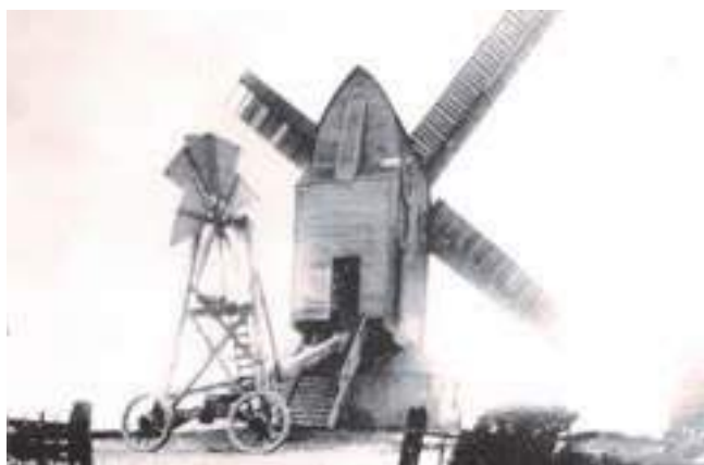
Fig. 2 Argos Hill Windmill c.1910 showing the unique cartwheels.
