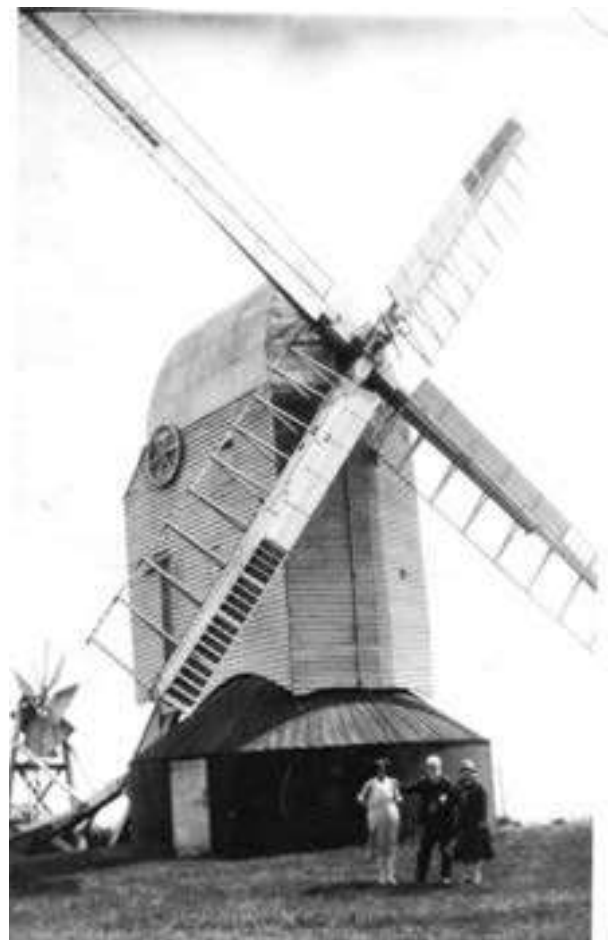
Fig. 1 Argos Hill Windmill in 1928, showing the sweeps with only the leading edge shutters in place. (from the Fuller family collection, by courtesy )
