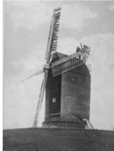
Fig. 8 Winchelsea Mill from a c1905 postcard published by A. H. Homewood, Burgess Hill. This shows one pair of common and one pair of spring sweeps.
