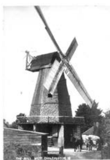
Fig. 10 West Chilmington Mill from a c1910 postcard published by F. Douglas Miller. This was a smock mill with balanced double shuttered spring sweeps.
