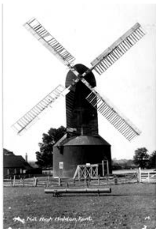
Fig. 5 High Halden Mill, Kent from a c1915 Wells Series postcard. Three of the spring sweeps are identical but the fourth is a later replacement.
