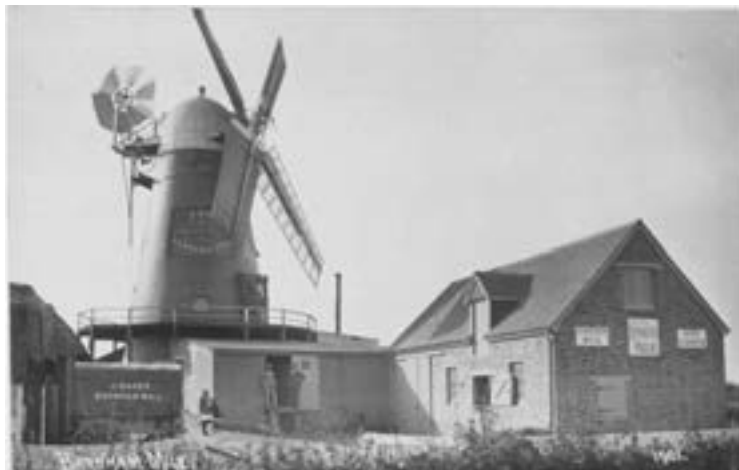
Fig. 10 West Chilmington Mill from a c1910 postcard published by F. Douglas Miller. This was a smock mill with balanced double shuttered spring sweeps.
