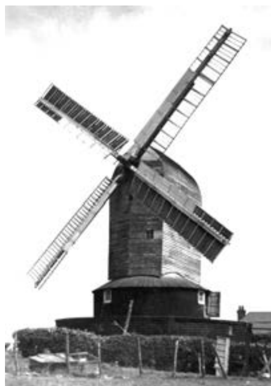
Fig. 6 Hoad's Mill, Bexhill from an undated postcard published by Wisemann Homer. Hoad's Mill was one of the group of mills with identical patent sweeps that stood in the Eastbourne/Hastings area.
