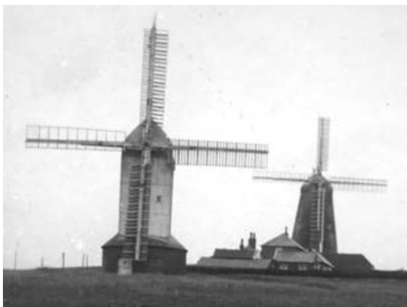
Fig. 4 Clayton Mills from a c.1900 photograph. Jill has unbalanced sweeps.
