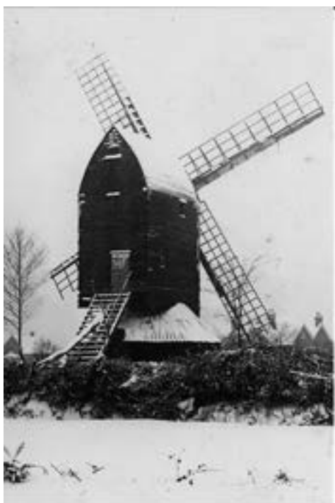
Fig. 3 North End Mill, East Grinstead, from a c.1890 photograph. The common sweeps are of an unbalanced design.
