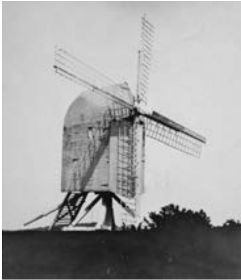
Fig. 7 Sullington Mill from a c1905 postcard showing the common sweeps typical of the area around Worthing.
