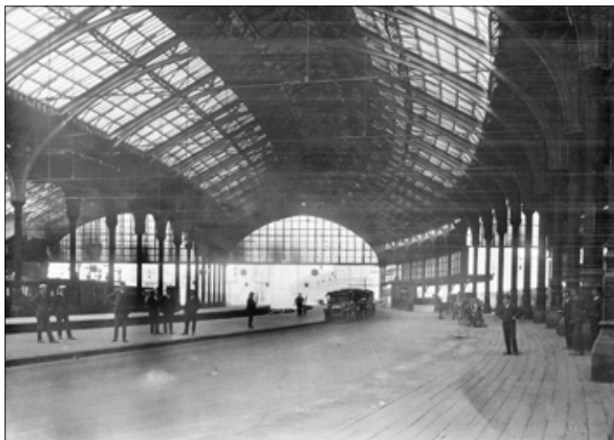
Exit of cab road into station. Note the horse cabs on one side and their motor replacement opposite which could not negotiate the hairpin bend. One of the columns on the right was supported by the box girder in the tunnel roof. See front cover (G F Burt)
