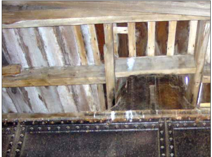
Box Girder support for one of the (1883) Train Shed roof support columns, this spanned the earlier Cab Road. (Martin Snow 2001)
