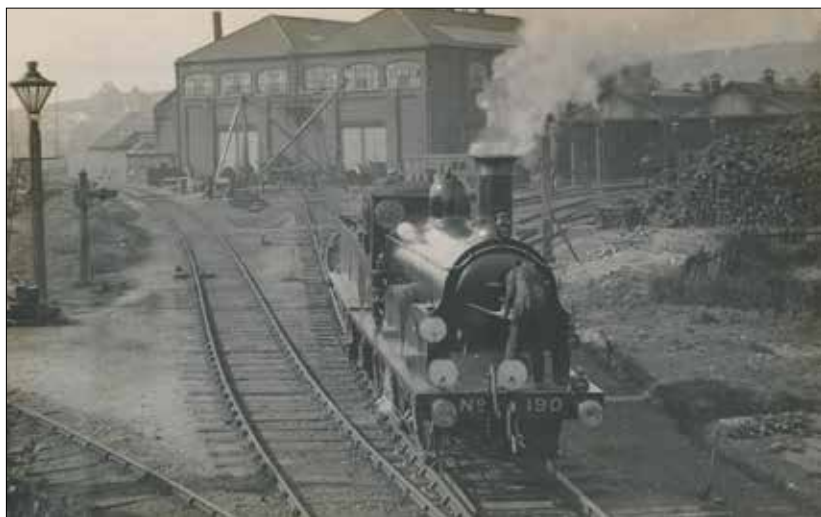
Works and shed c 1900
