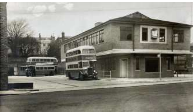
Fig. 1 A view of Lewes Bus Station from Eastgate Street in the early 1950s which clearly shows how the overhanging upper storey provided shelter for waiting passengers. Sadly the projecting clock and Southdown lettering have disappeared, having been replaced by an advertisement hoarding. Southdown 254 (GCD 354) a 1939 Leyland TD5 re-bodied by Northern Counties in 1950, waits to depart on service 28 to the Landport Estate. Another TD5, this time re-bodied by Park Royal, lurks in the background. To the left of the picture can be seen the east wall of the garage.
