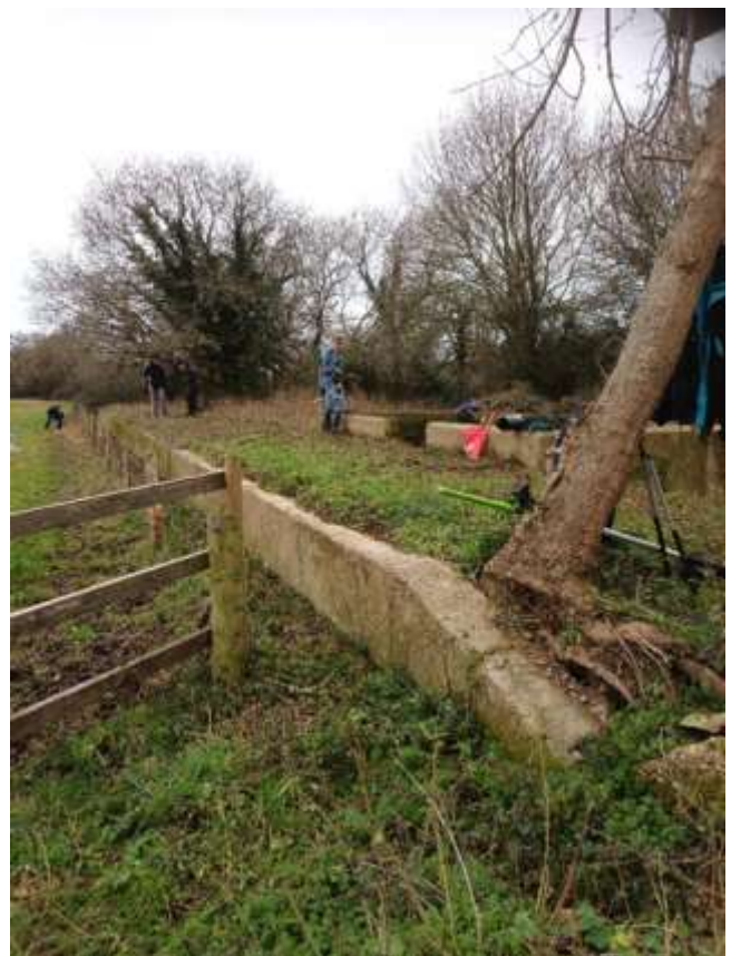
Fig. 7 Chalder Station Platform and the base of the Waiting Room
