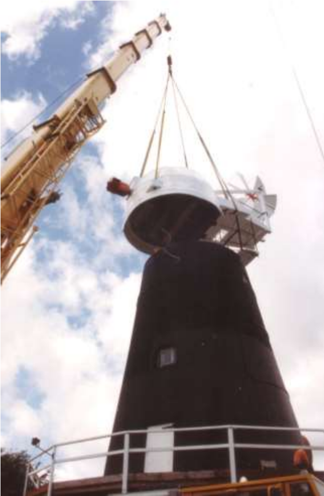
Fig. 4 Raising the new cap by crane, June 1999.
