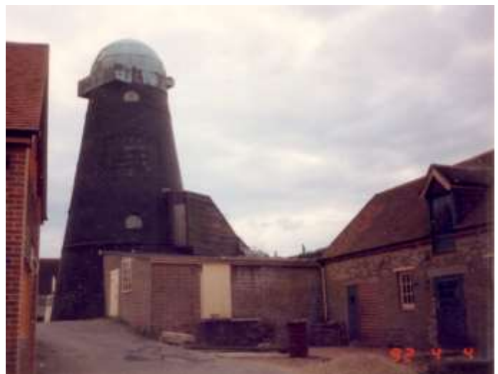
Fig. 3 Barnham Mill prior to renovation, 1992
