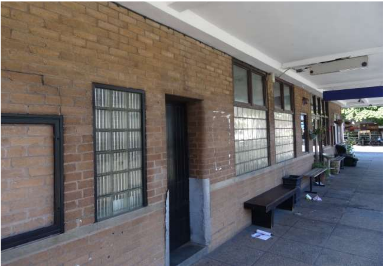
Fig. 3 A view under the overhang on the west side of the bus station in June 2022 shewing the glass-block windows. The bus station was still in use and the cafe open for business – but not for much longer ( Author )
