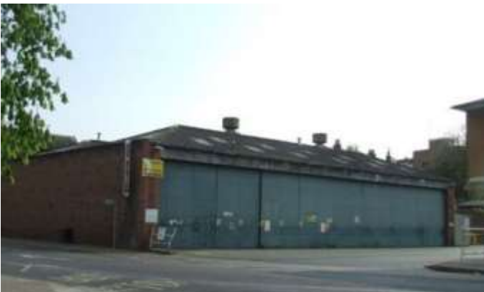
Fig. 4 The north elevation of the bus garage seen after it had been taken out of use. The prominent ventilators to remove exhaust fumes can clearly be seen. The vertical white 'Bus Station' sign on the wall was to direct those approaching from Friars Walk as the view of said bus station was eclipsed by the garage.
