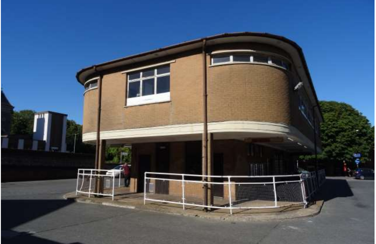
Fig. 2 The rear of the bus station was seldom photographed, but here it is seen in June 2022 when the threat of imminent closure was hanging over it. It shews the radiused corners and the slender columns supporting the first floor ( Author )
