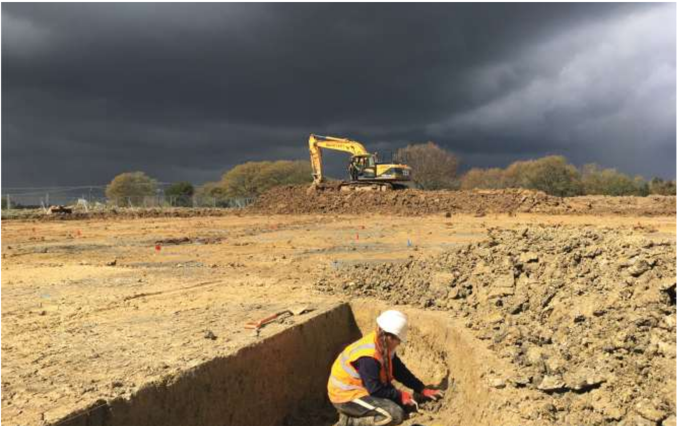
Fig. 3: Photograph of a Horam minepit during excavation
