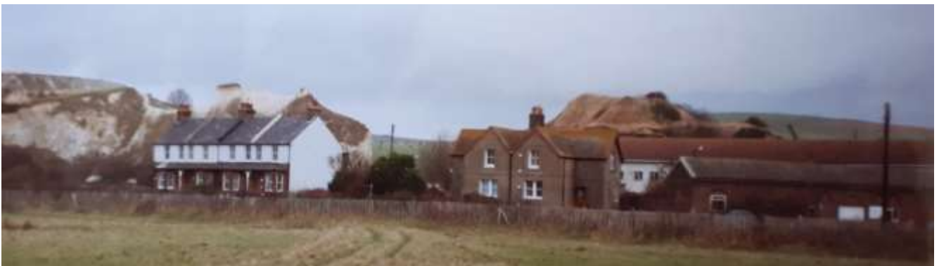
Fig 4. Works Cottages to the left and Stable Cottages to the right in 1993. The long low building extreme right is the work's stable block. The building behind the stables is an industrial unit no longer (2022) in existence.
