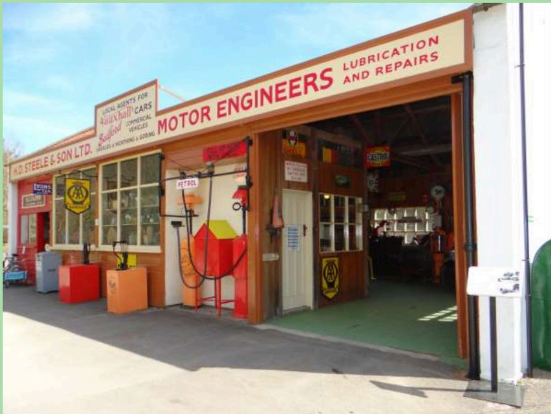
The Village Garage at Amberley Museum, a replica of a typical building of the 1920s/30s
