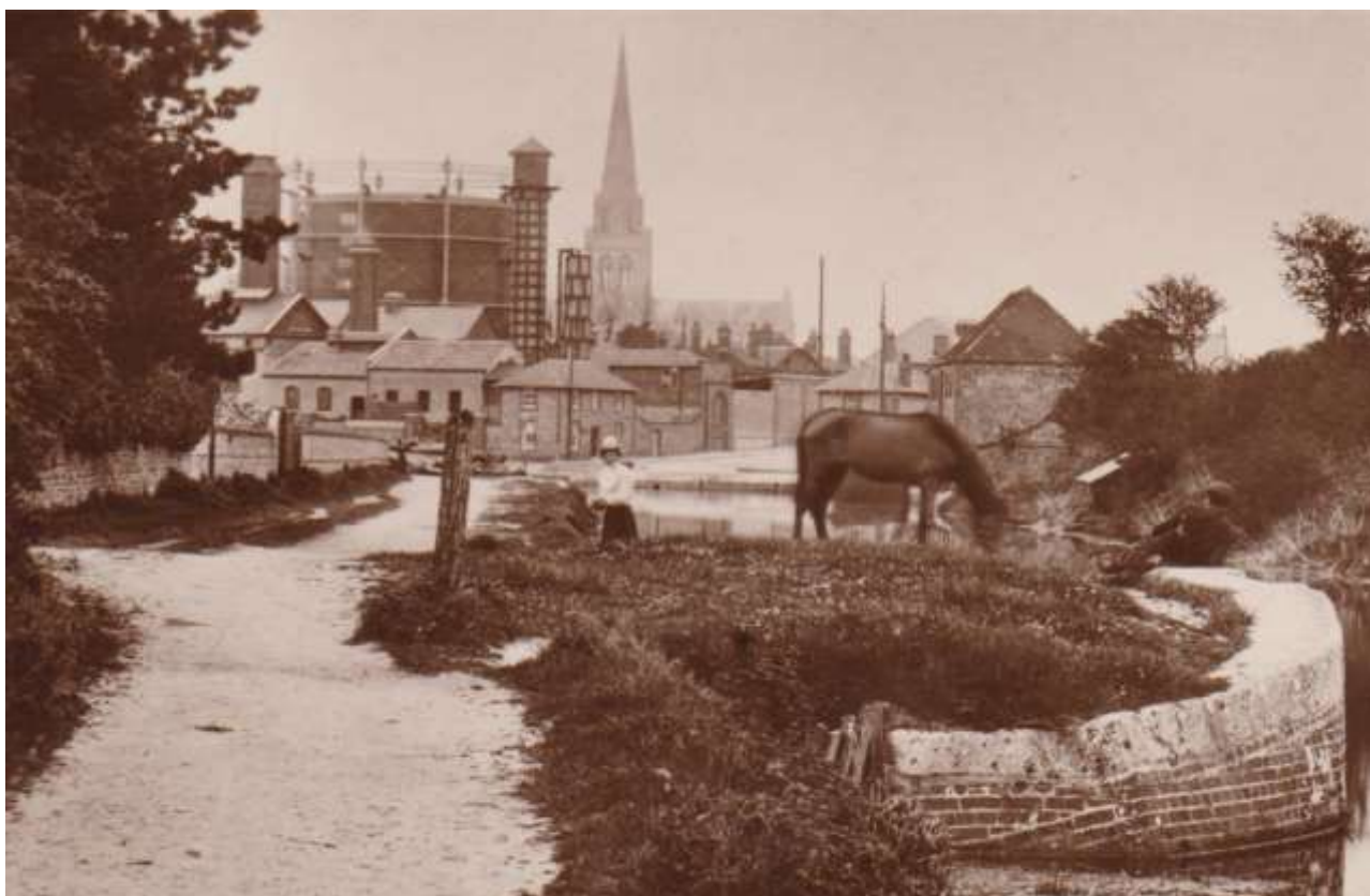
Fig 7. A view of Chichester looking north from the canal with the enlarged gasworks in the middle ground. To the left is the chimney of the retort house and to the right the two towers are the scrubbers which wash ammonia out of the gas. One of the gasholders provides the back drop. (Author's collection)
