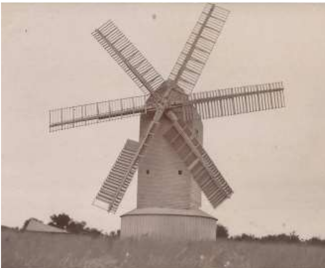
Fig 10. Ashcombe windmill and a partially collapsed out-building in c1910. The shutter lengths have been modified from the original configuration.
