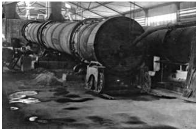
Fig 4. The Shoreham kilns, believed to be identical to the one installed at Newhaven in c.1901/2 (Photo courtesy Dylan Moore, www.cemenkilns.co.uk )
