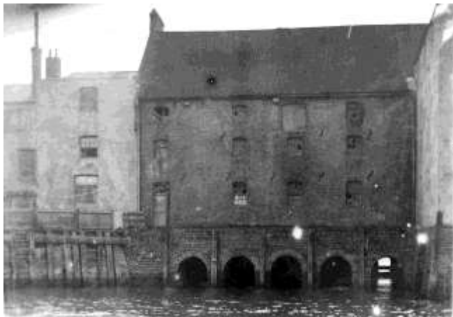
Fig 11. West elevation of original Tide mill showing loading door and gantry (courtesy Seaford Museum)
