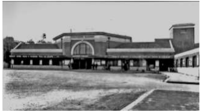
Fig. 4. The frontage of Robb Scott's Hastings station as built. The Diocletian window imparts an element of neo-classicism. The square tower to the right is one of the luggage lifts. Note the enamel signs attached to the canopy vaunting the express services on offer. 'Express' has to be interpreted as a relative term as far as the services to the north were concerned. ( Railway Station Photographs )
