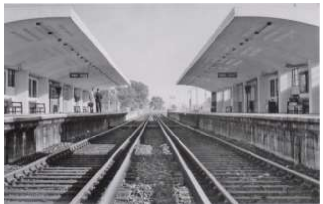
Fig. 3 Chessington North on the Chessington Branch, opened in 1939, is perhaps the most bold of Robb Scott's designs with its white-painted curvilinear, reinforced concrete cantilevered canopies, and horizontal Crittall windows set in the back walls. (Author's collection)
