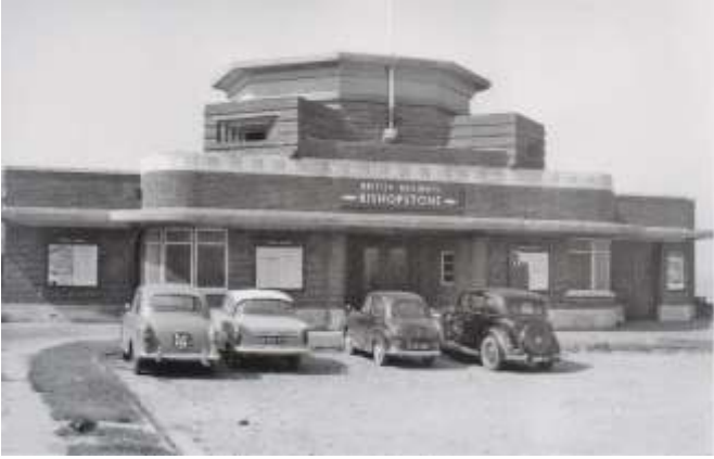
Fig 15. The frontage of Bishopstone in BR days. The two pill boxes added later to the roof look as though they had been intended as part of the original design. Note the flagpole and compare the actual fenestration with the architect's drawing in Fig 14 above. The view has little changed today but the vast numbers of cars now parked here makes photography very difficult. ( Author's collection )
