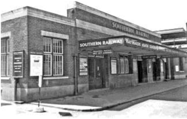
Fig 8. The frontage of Haywards Heath in early BR days shewing the rather plain building with its wide canopy.
