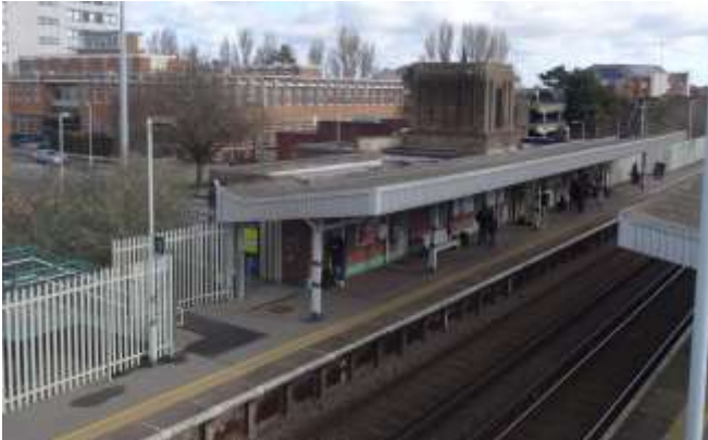
Fig 13. The up platform viewed from the footbridge. The canopies have been re-clad in 'crinkly tin' and the door on the front of the tower can be seen! (Author)
