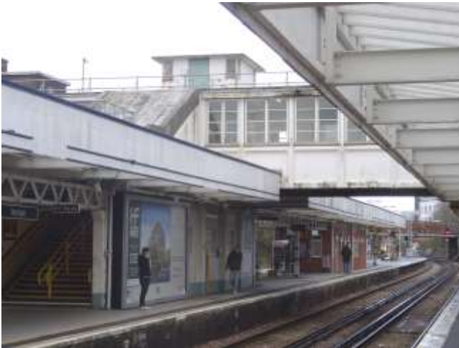
Fig 20. A view of the up platform looking towards London showing the standard steel canopies, concrete footbridge and platform buildings. The square structure on top of the bridge is one of the luggage lifts. (Author).
