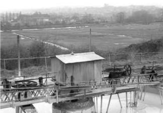
Fig. 5 Slurry storage tank
