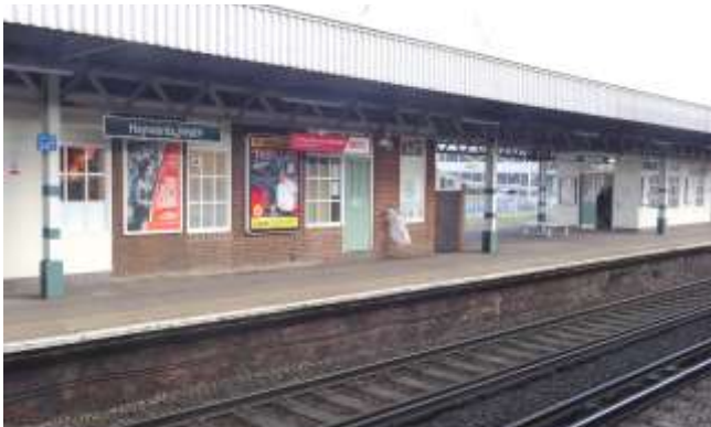
Fig 9. The down platform buildings today which are a mixture of timber and brick construction beneath a standard SR steel island platform canopy supported on a double row of columns. Note that instead of Crittall steel windows multi-paned timber lights have been provided. ( Author )
