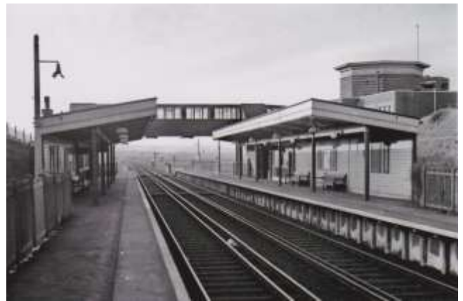
Fig 16. Bishopstone viewed from the up platform in the 1960s looking towards Newhaven. The elevation of the building above the platforms can be appreciated here. The canopies are of steel and carried on rolled steel columns but there are no facilities at platform level. Other typical SR details to note are the octagonal lampshades under the canopies and the concrete lampposts. The down (far) platform was taken out of use in 1975 and its canopy demolished. ( Ben Brookshank )
