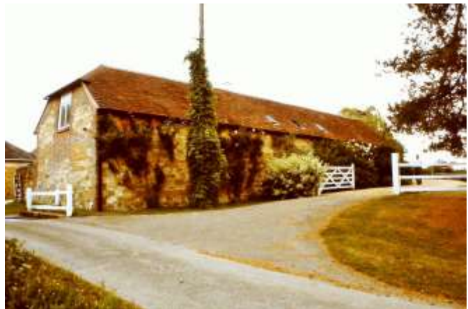
Fig.8 Fisher Street Malthouse
