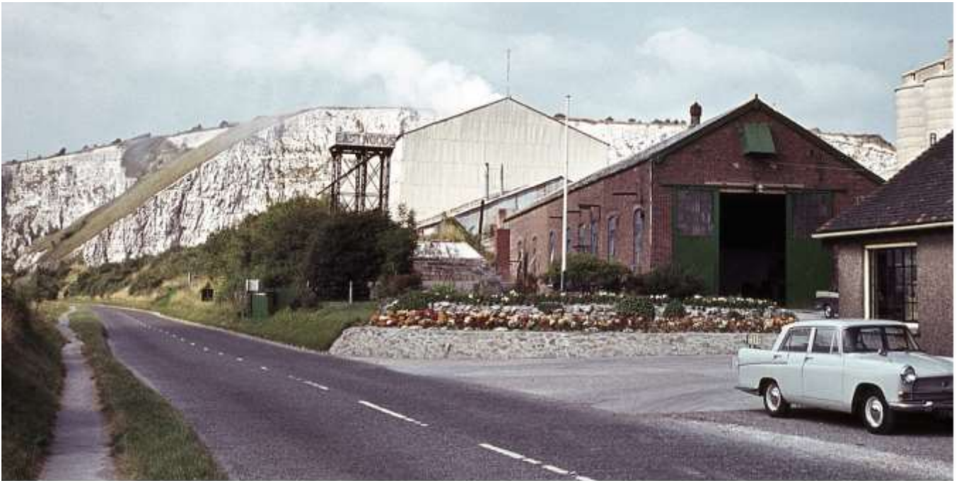
Fig. 1 Southerham Cement Works, 1964
