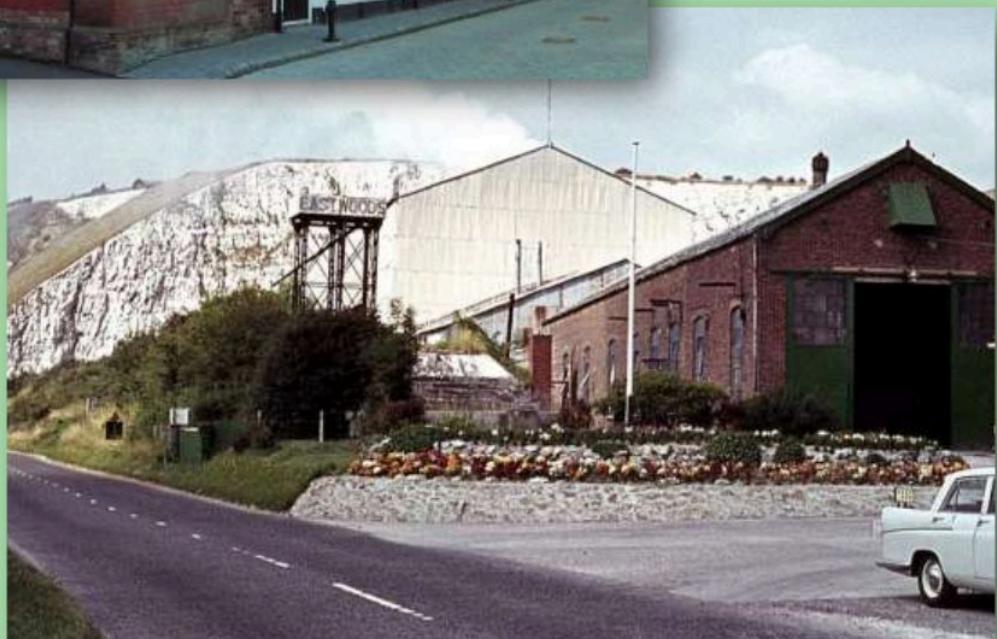
Southerham Cement Works, 1964
