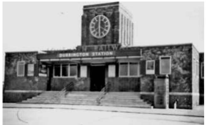
Fig 12. The frontage of Durrington-on-Sea as built, shewing the central tower with its massive clock face and the wide flight of steps to the entrance. No concessions were made to disabled access in 1937! Sadly the clock and the Southern Railway lettering have gone, and the original Crittall windows have been replaced in plastic. (Railway Station Photographs)
