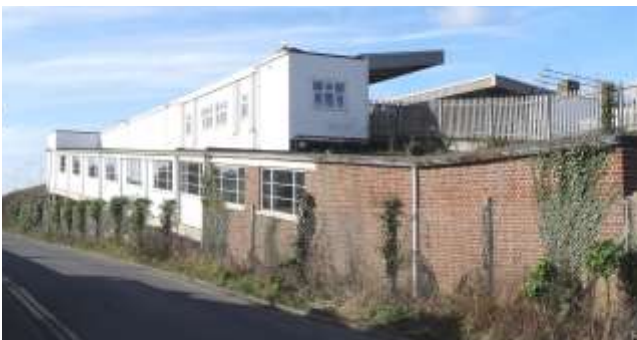
Fig 11. The up platform viewed from road level shewing the covered ramp whose construction starts off in brick but soon becomes concrete framed with timber infill, and also the timber platform screen. (Author)
