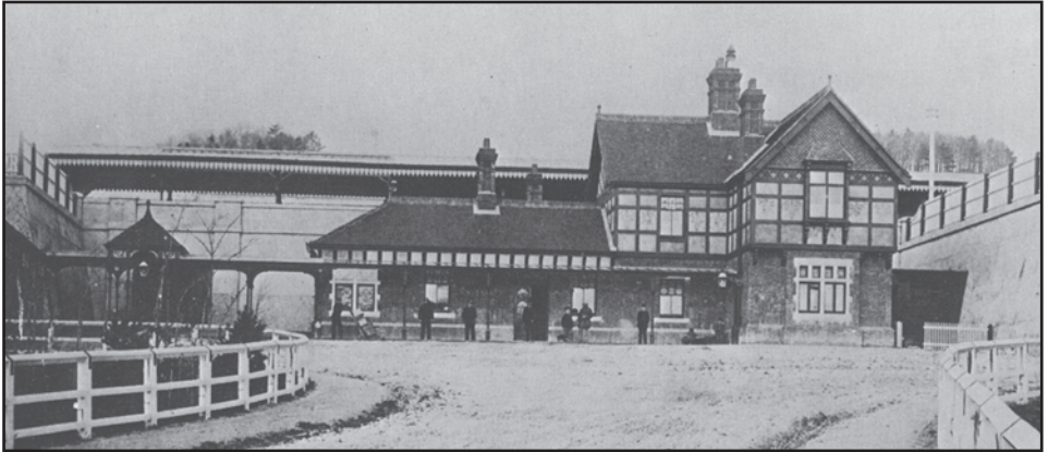
The frontage of Singleton taken from an album of photographs produced in 1881 for Frederick Banister, the LB&SCR Chief Civil Engineer.
