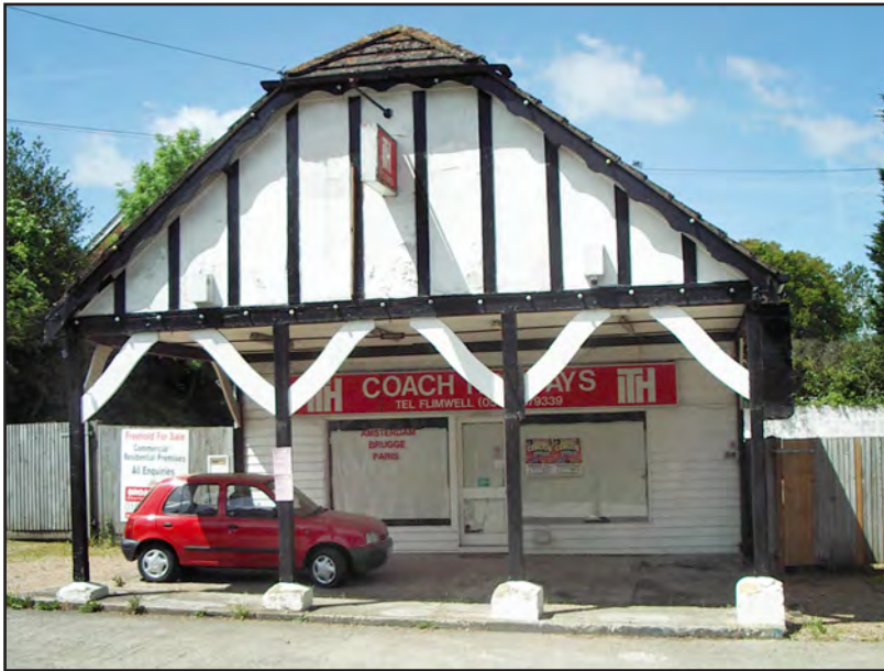
Former garage at Flimwell, Ticehurst, East Sussex. Recently listed as part of the English Heritage Cars Project. (Peter Holtham)
