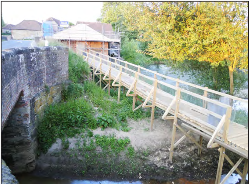
Progress with the new boardwalk, part of the development at Coultershaw. Visitors will be able to use the boardwalk to access the former lock on the Rother Navigation that now has a footpath laid through it. (Martin Snow)
