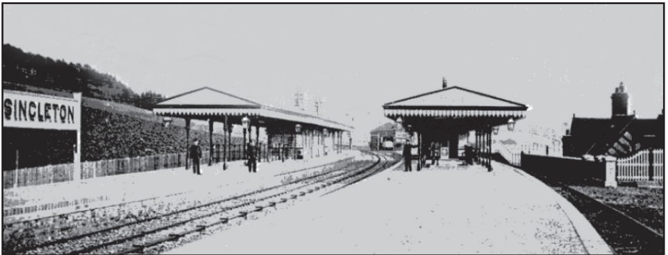
Another view from Frederick Banister's 1881 album, this time showing the two island platforms at Singleton looking towards Midhurst. The canopies here have gabled, rather than hipped, ends. The goods shed can be seen in the centre background. (WSRO)
