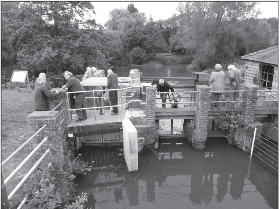
Members viewing the Archimedes screw turbine (left) and sluices at Coultershaw, taken from the road bridge. The original watermill waterwheel was to the left, when the old turbine was installed for the mill the wall at the left was built and rubble dumped in the gap, this had to be stabilised for the new turbine. The engine house is just visible on the right, the power shafts to the mill ran across the top of the sluices. (Malcolm Dawes)
