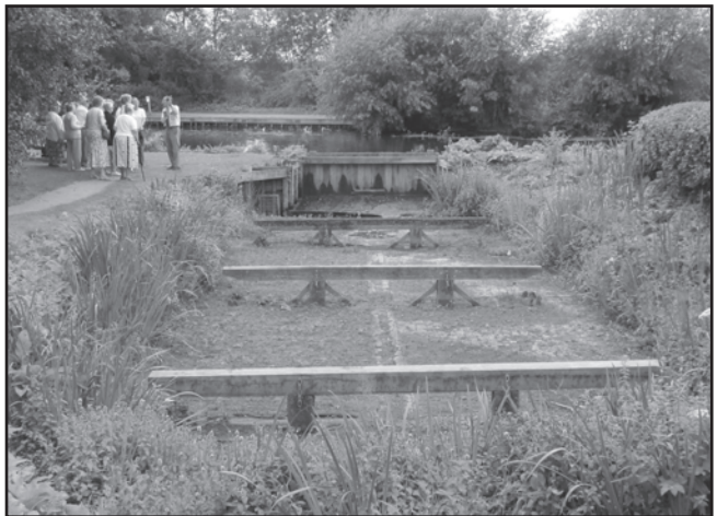
The restored dry dock, featured by John Constable. (Ron Martin)
