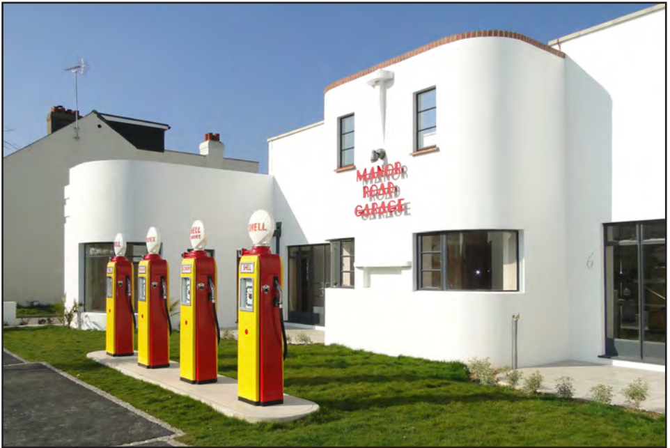
The former garage in Manor Road, East Preston, March 2012. Compare this new view to that on the cover of Newsletter 140 . The petrol pumps have been restored to pristine appearance and the garage converted to housing. It is pleasing to see a sympathetic conversion of the front of this Art Deco survivor. ( Martin Snow )
