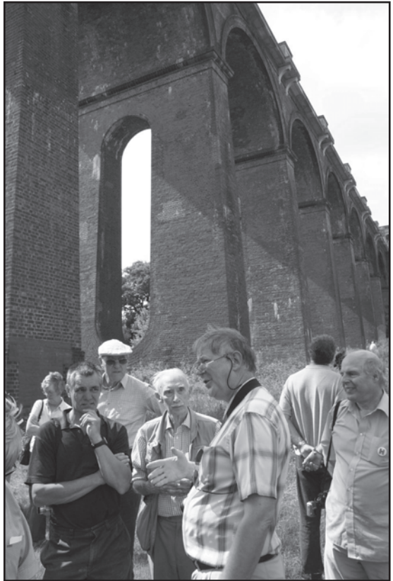
Alan Green detailing the Ouse Viaduct to assembled members - who's that with the Heritage badge?
