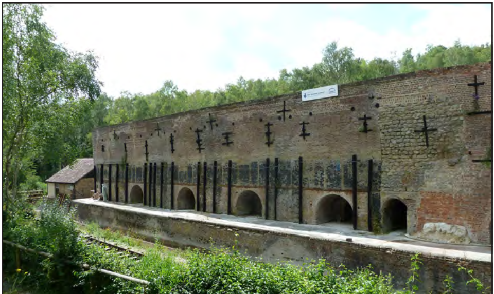
The newly restored DeWitt Kiln block at Amberley Museum.
