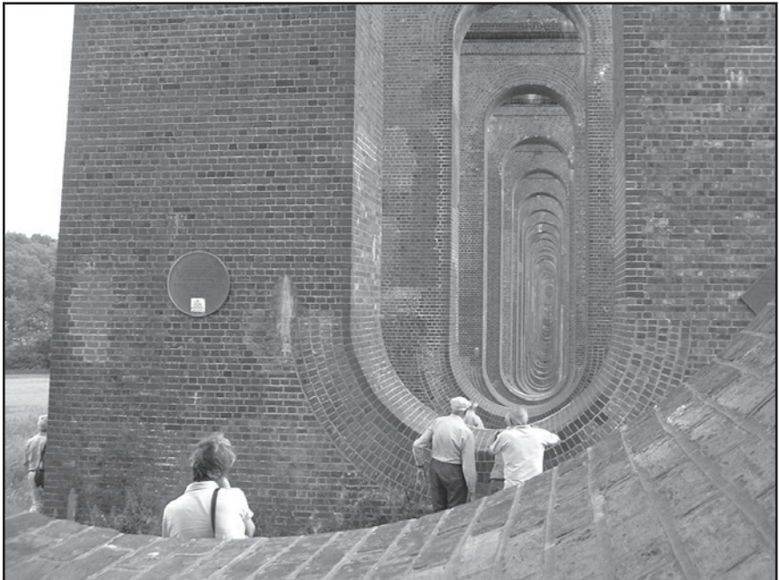
Members viewing the long line of brick arches
