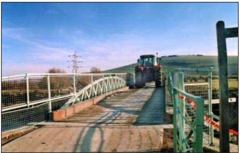
The 'first' tractor passes over the reopened Southease bridge. In actual fact the bridge had been brought back into use a few weeks earlier! The new weldmesh screens to the papapets can be seen, as well as the new timber decking. (*Alan Green*)
