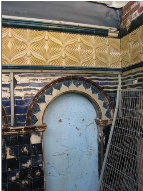
Faience slabs, Medina House, Hove ( Ron Martin )
