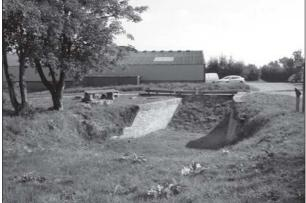
Hollinsworth Bridge Showing the infilled canal bed at site of bridge with curved retaining walls
