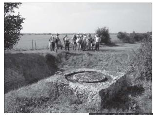
Block with groove for lower part of ball race of bridge bearing
