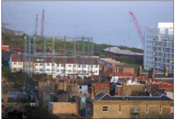
Black Rock gasworks 2021
