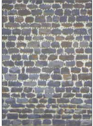
Selbourne wall with ‘tenpenny nails’
