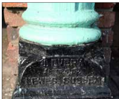
Madeira Terrace arches rainwater spout displaying foundry details
