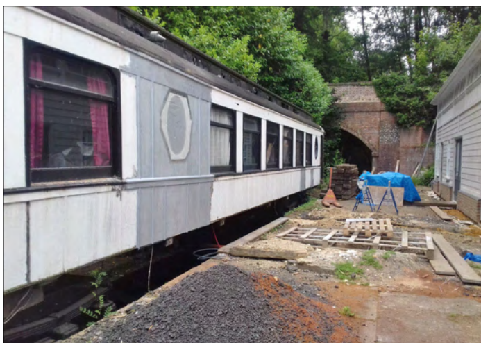
Princess Ena and building site
