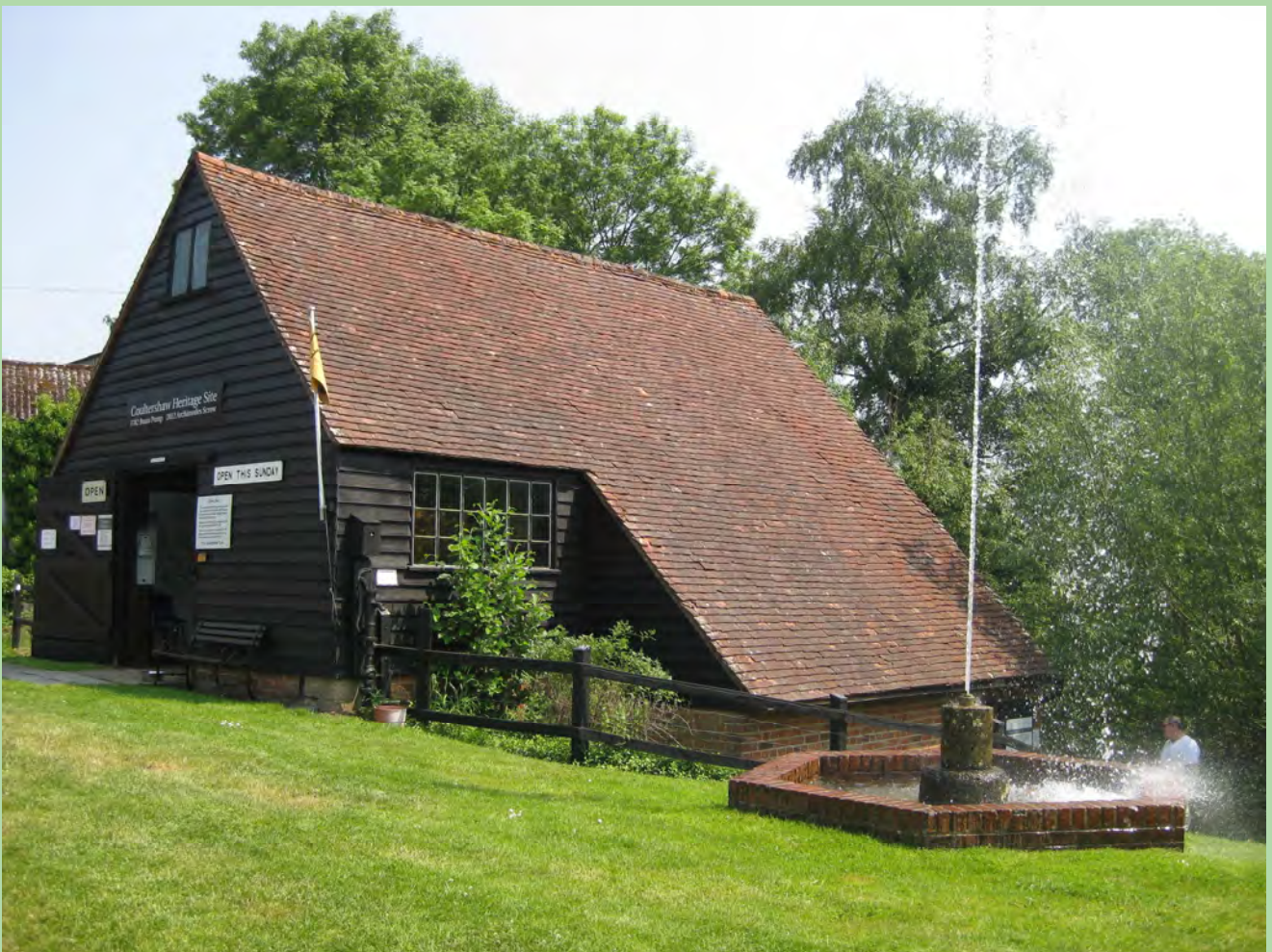
Coultershaw Beam Pump—pump house and fountain
