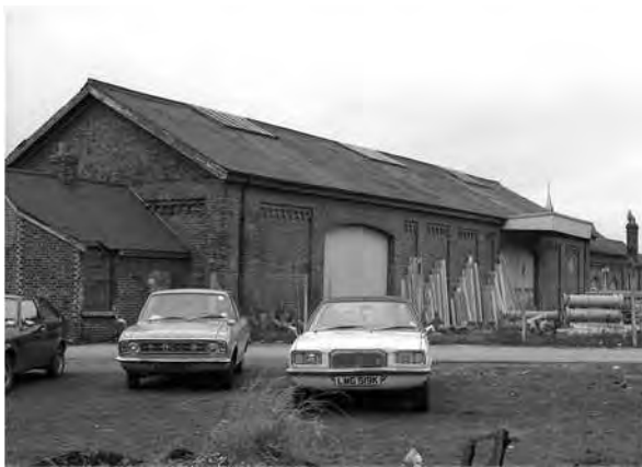
Fig. 10 The 1846 goods shed at Lewes, originally entered via a wagon turntable at the side. Photographed 1980. John Minnis
