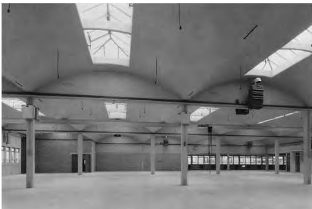
Fig. 2 Standard unit 'wavy roof construction: Above: exterior Below: interior (Crompton Way)
