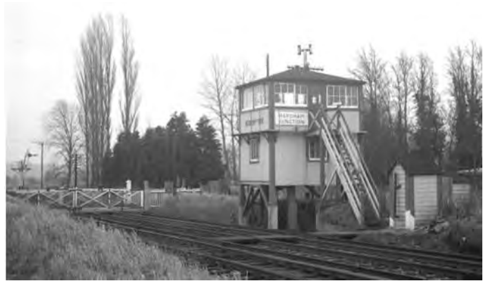
Fig. 11 A loss of national significance in the history of railway signalling was Hardham Junction signal box. Built in 1863, it was the last survivor of the original design of box introduced by John Saxby in 1858 with the operating floor mounted high off the ground on large baulks of timber, providing a good range of vision for the signalman. Seen here on 2 February 1967, it closed on 21 March the same year.
