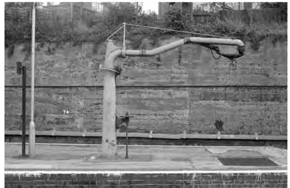
Fig. 15 Stroudley pattern water column from the 1880s at Lewes, 20 August 1970. John Minnis
