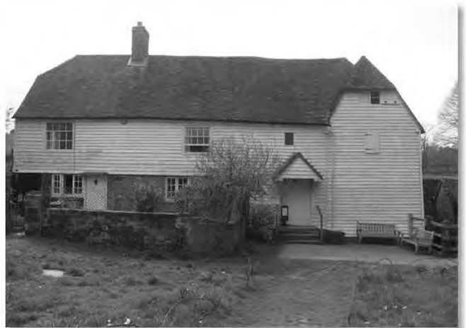
Fig. 16 Park Mill at Batemans, Burwash, restored, April 2014 (Photo by Philip Hicks)
