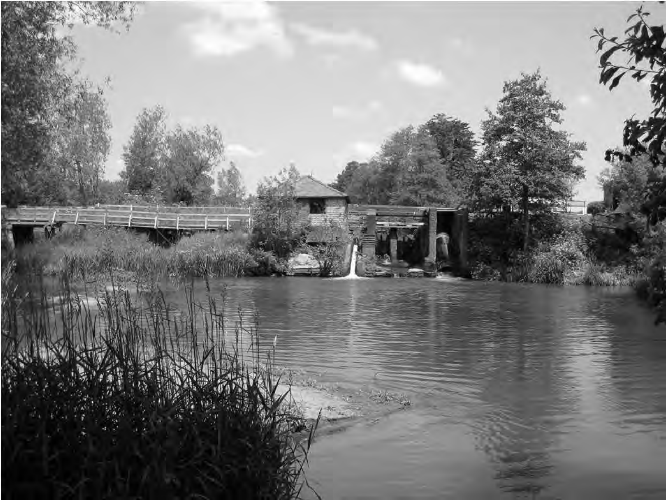
Fig. 8 View across the Mill Pond showing the second boardwalk constructed at a higher level, refurbished engine house, fish ladder, two sluice gates and Archimedes Screw.
