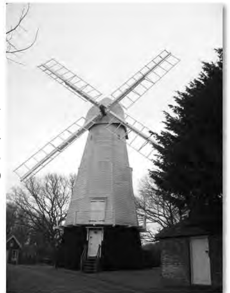
Fig. 10 Chailey Mill restored, March 2017 (Photo by Philip Hicks)
