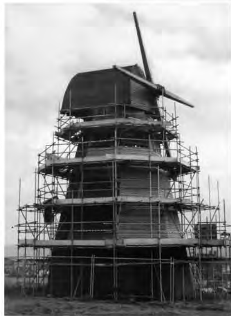
Fig. 11 Rottingdean Mill during renovation work in September 1999 (Photo by Philip Hicks)
