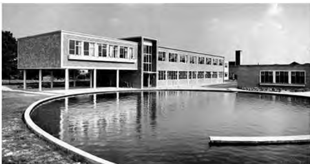
Fig. 16 Telcon Metals ( West Sussex Past Pictures )
