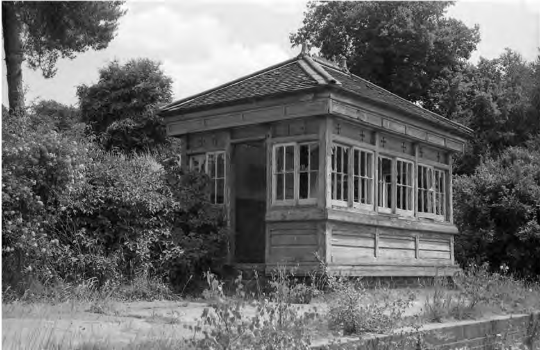
Fig. 13 Most signal boxes were constructed to standard patterns but T H Myres designed a special box to accompany his Domestic Revival stations, employing tiled rather than slated roofs, ornamental terracotta ridge tiles, boxed eaves and quatrefoil motifs in panels above the windows. The result was one of the most handsome signal box designs of which just one example, at Horsted Keynes, survives. This is Midhurst East of 1881, closed in 1925, but retained as an office, and photographed while derelict on 17 July 1969 before demolition later that year. John Minnis
