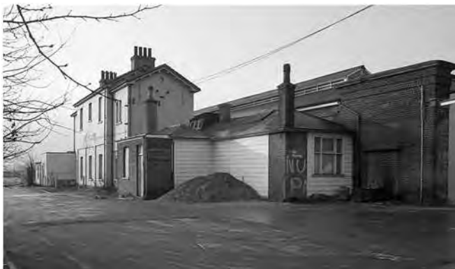
Fig. 1 Three Bridges in May 1980. The 1841 Mocatta station building on the down side, with the upper floor subsequently added to provide accommodation for the station master. The Italianate detailing closely resembles that at Hassocks.
