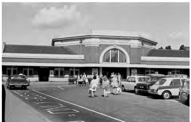
Fig. 6 Hastings, a handsome structure of 1931 by the SR's architect, J R Scott. Photographed 20 August 1970. John Minnis
