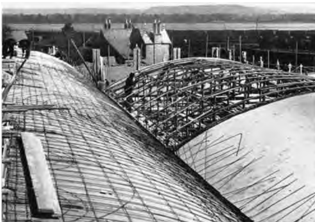
Fig. 2 Standard unit 'wavy roof construction: Above: exterior Below: interior (Crompton Way)
