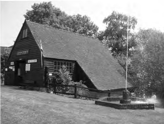
Fig. 4 Exterior of pump house, showing the fountain.
