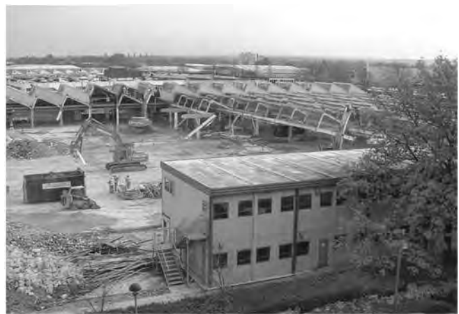
Fig. 7 The demolition of Edwards High Vacuum
