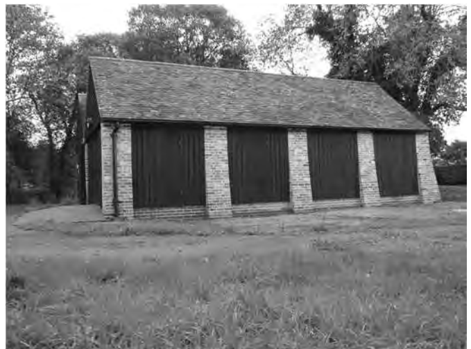
Fig. 6b Warehouse restored in 2013.
