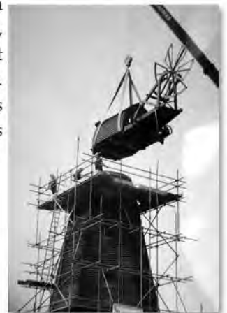
Fig. 8a West Blatchington Mill. Lifting the newly restored cap back onto the tower, 1999 (top).
