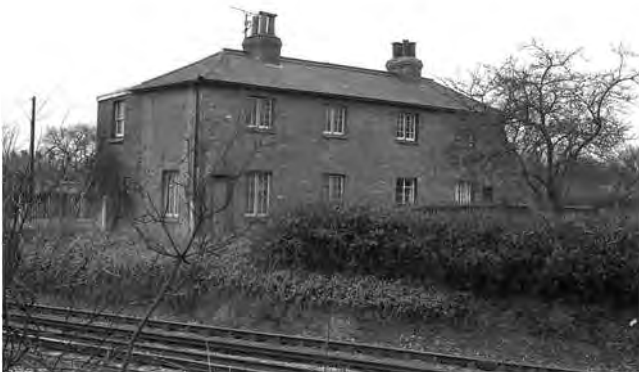
Fig. 14 Railway cottages at Keymer Junction, built in 1850 at a cost of £237, were good examples of the relatively small buildings put up at that time for the company's staff. Photographed April 1983. John Minnis
