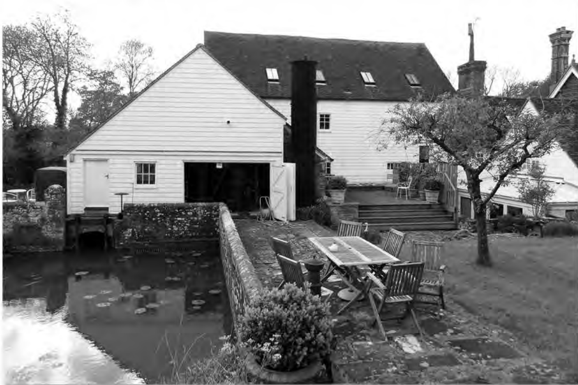
Fig. 19 Cobbs Mill at Hurstpierpoint, house-converted but retaining much of the machinery, 2014 (Photo by Philip Hicks)
