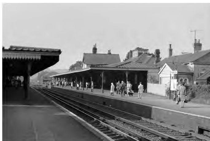
Fig. 2 Hassocks. T H Myres' station was the largest of his Domestic Revival designs and replaced the Mocatta building seen on the right, which was retained as staff accommodation. John Hoare/SIAS
