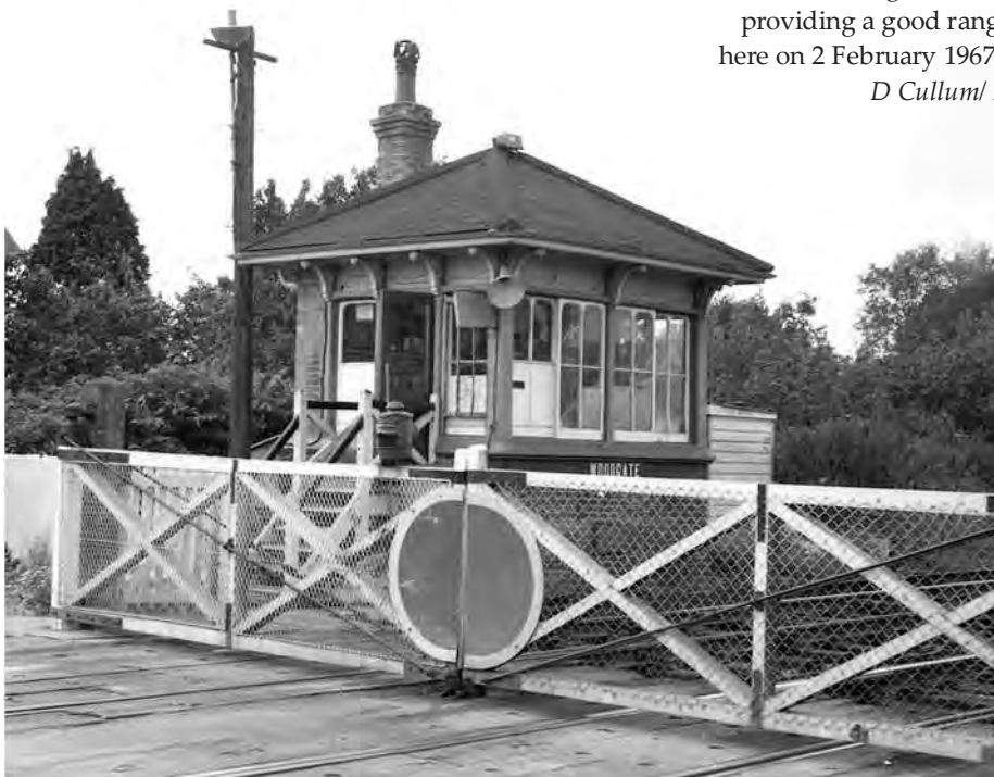
Fig. 12 Woodgate serves as an example of the many boxes of the Saxby & Farmer type 5 design used on the LB&SCR. Built in 1876 and closed in 1985, it retained an LB&SCR nameboard when photographed in 1971. The gates are another feature that, with the removal of those at Plumpton, is almost extinct in the county. John Minnis
