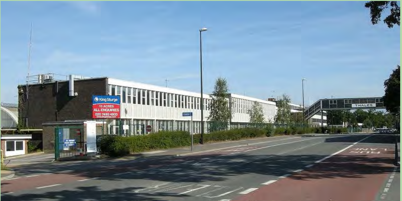
Redifon/Thales factory in Gatwick Road, Crawley, prior to demolition in 2011 (copyright Anthony Rouse)
