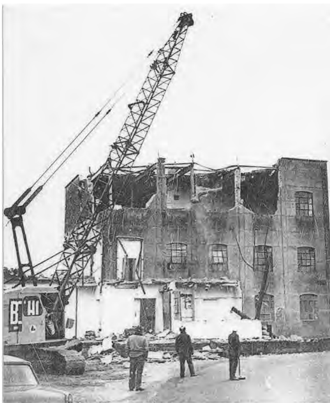
Fig. 1 Demolition of the former concrete Coultershaw Mill in 1973
