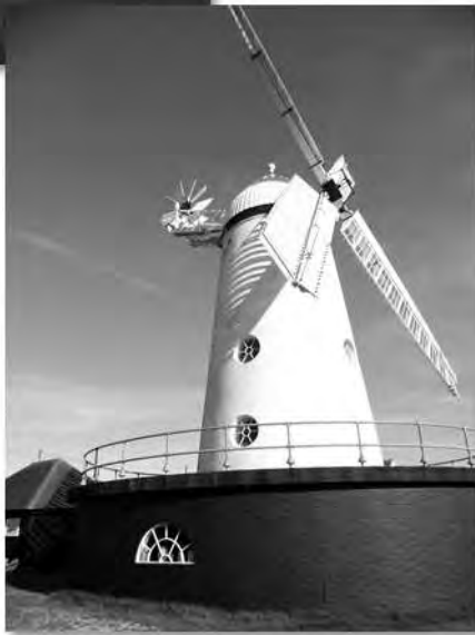
Fig. 7b Stone Cross Mill in working order, March 2017 (Photo by Philip Hicks)
