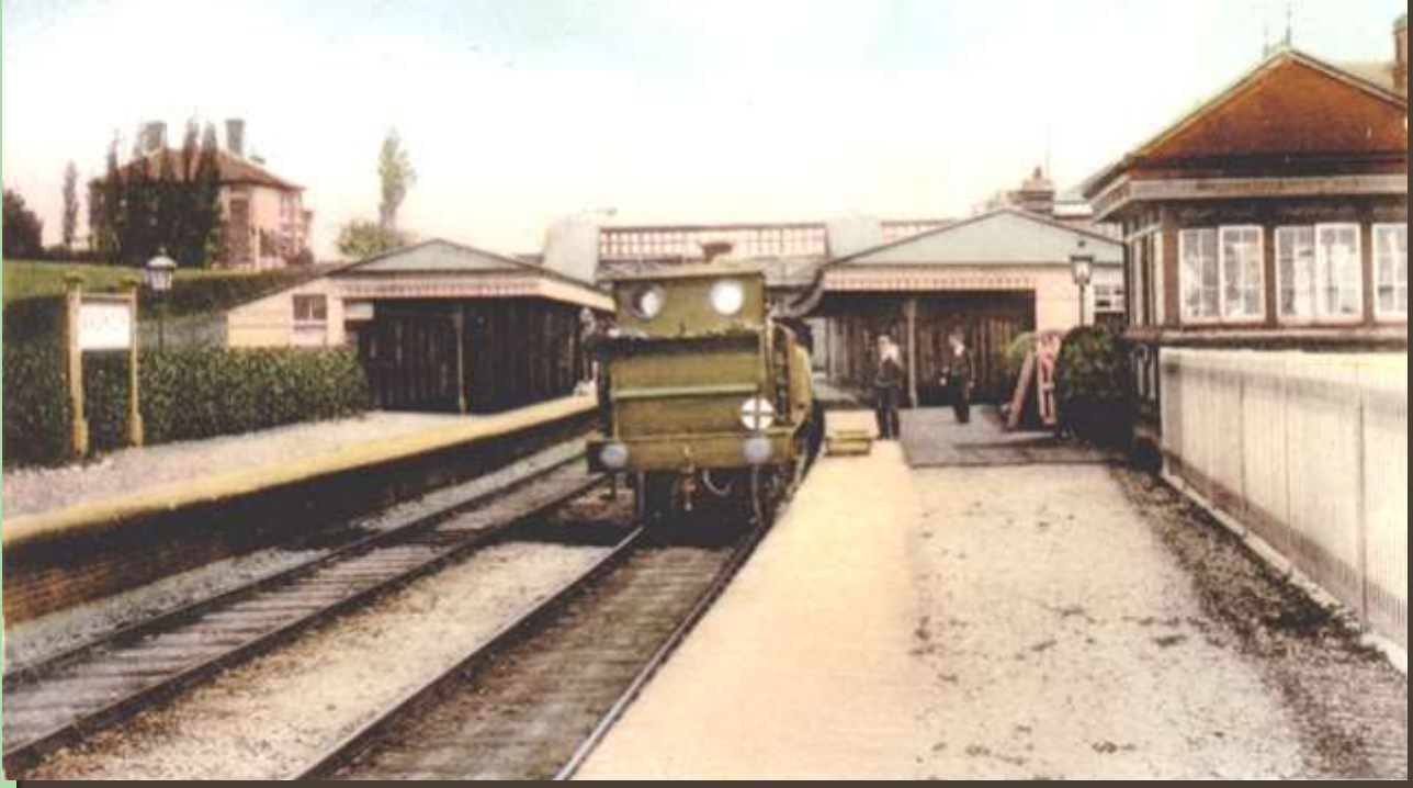
A postcard view of the frontage of Ardingly station in pre-grouping days showing a T H Myres building in original condition with its mock timbering and pargetting which have since been lost. The exceptionally lofty chimney pot is worthy of note. (Alan Green collection)
