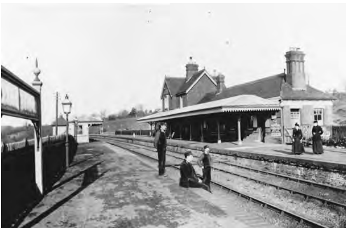
Fig 6. Rotherfield & Mark Cross, also on the Cuckoo line, seen in pre-grouping days. This is a Type 'B' station with the extended single storey section nearest the camera containing a refreshment room. (Author's collection)
