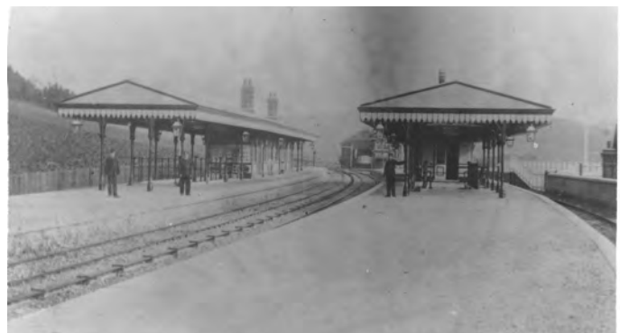
Fig 10. Another view from Frederick Banister's 1881 album, this time shewing the two island platforms at Singleton looking towards Midhurst. The canopies here have gabled, rather than hipped, ends. The north signal box and the goods shed can be seen in the centre background. (WSRO)
