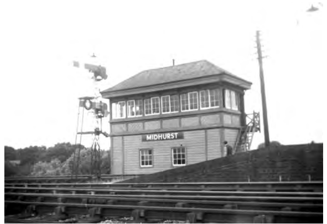
Fig 18 The main signal box at Midhurst (originally 'Midhurst North') was all of timber, possibly to reduce the loading on the weak embankment, but the detailing is characteristic Myres. The former south box was on the up platform and, after decommissioning, saw further service as the station master's office. (Author's collection)
