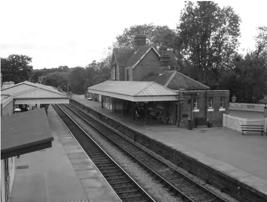
Fig 21. Sheffield Park (Type 'A') looking north in July 2015. The canopies, which had been drastically shortened by the Southern Railway, have been returned to their full length and the elaborate valances, which were unique to the Bluebell Line, have been recreated by BRPS. With its LB&SCR colours, Sheffield Park is very much in pre-grouping form – only the timber foot bridge is lacking. (Author)
