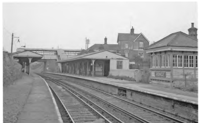
Fig 8. Ardingly in BR days looking towards Horsted Keynes. The station buildings can be seen at high level at right angles to the track and connected to the platforms via a timber footbridge. The canopies have gabled rather than the usual hipped ends. The platform-mounted signal box was also designed by Myres. Although the building still exists at road level, everything at track level has been destroyed. (Author's collection)
