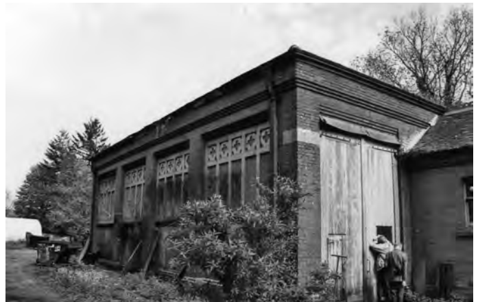
Fig 19. Singleton goods shed being examined by SIAS members on the occasion of the Society's visit on 3 May 2008. This shows the north (track) side of the building with the characteristic Myres mock-timbering and pargetting. The goods office is to the right. (Author)
