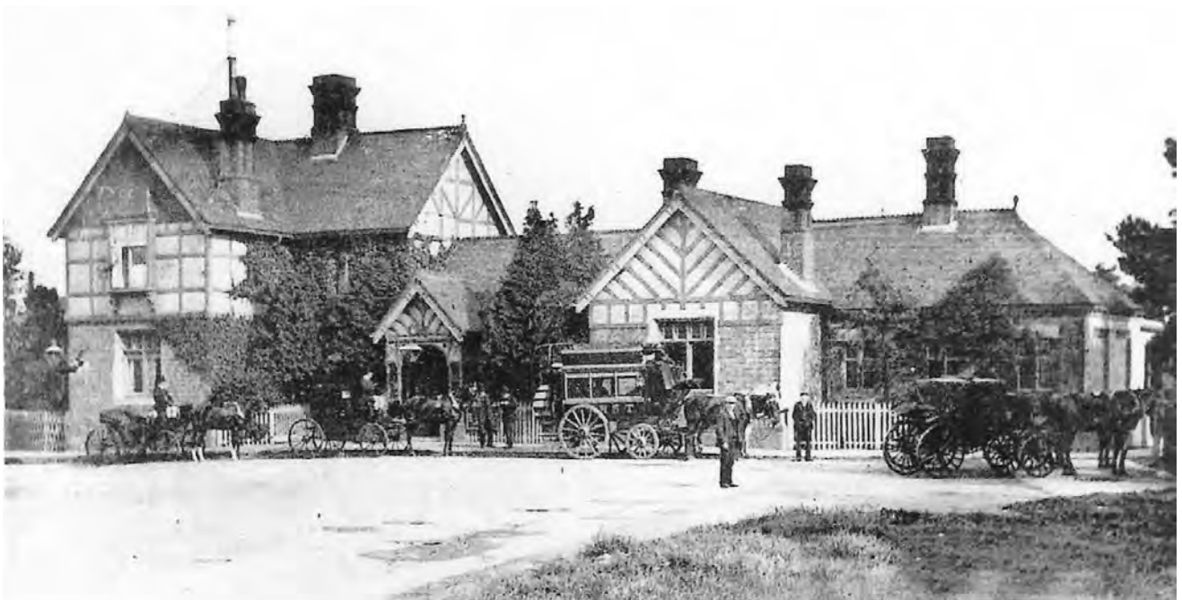
Fig 2. A pre-grouping view of the frontage of the upside buildings at Hassocks which makes an interesting comparison with Ardingly (see Fig 1). The gabled transept to the 'business' section of the building housing the refreshment room was not repeated on later versions and the pattern of the mock timbering also changed. The timbering here was later removed but the walls were not tile hung as happened elsewhere. Hassocks is still open but all the Myres buildings were destroyed in the 1970s. (Author's collection)
