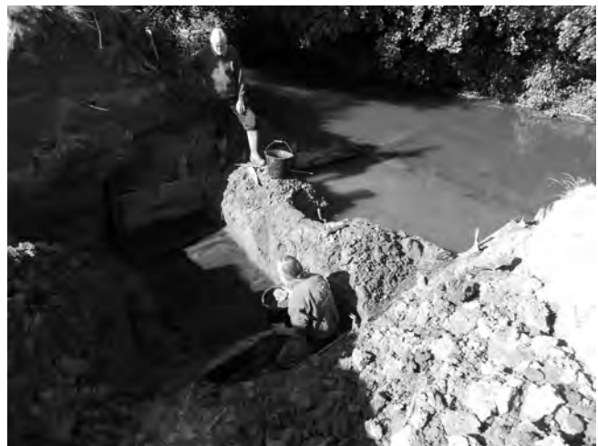
Fig 6 (above). The boarding, side planks and upright posts exposed. The centre bulk remains to hold the river back. Gordon Hall is seen sponge cleaning the boards with the writer looking after bailing out.
