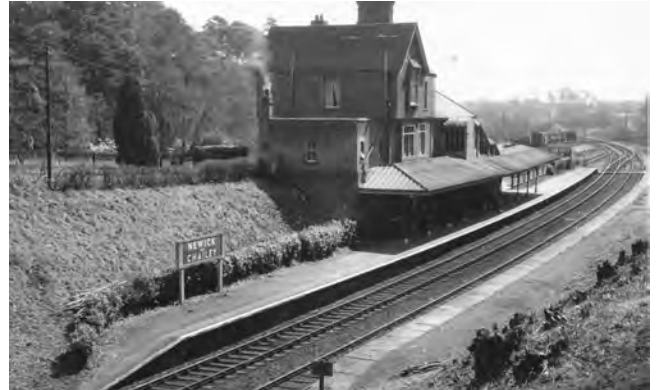
Fig 7. Newick and Chailey looking towards Barcombe. This shows the three-storey platform-side elevation of a Type 'C' station. At this time the up platform was out of use and the waiting shelter and footbridge had been demolished. The stairs of the footbridge are still in situ on the down platform though, giving access from the first floor booking office. It can be seen how the approach road in the background is at first floor level. (Author's collection)
