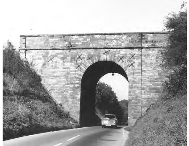
Fig 9. Flyover at the Harrow
