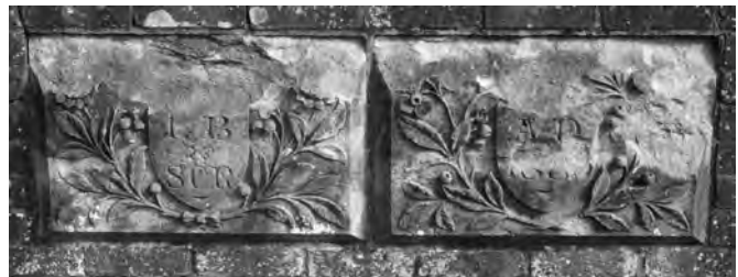
Fig 15.(Left) Cartouches over the ladies' lavatory window at Midhurst displaying the company ownership and the year of construction. These stone mullioned lavatory windows were a standard Myres detail, but on Cuckoo line stations the panels were left blank whilst on the Bluebell line an LB&SCR monogram and the date - 1882- were displayed in cursive characters. (Right) on demolition of Midhurst the cartouches were set into a new wall in the housing estate and survive today, albeit damaged, as the only reminder of the once fine station that occupied the site. (Author)
