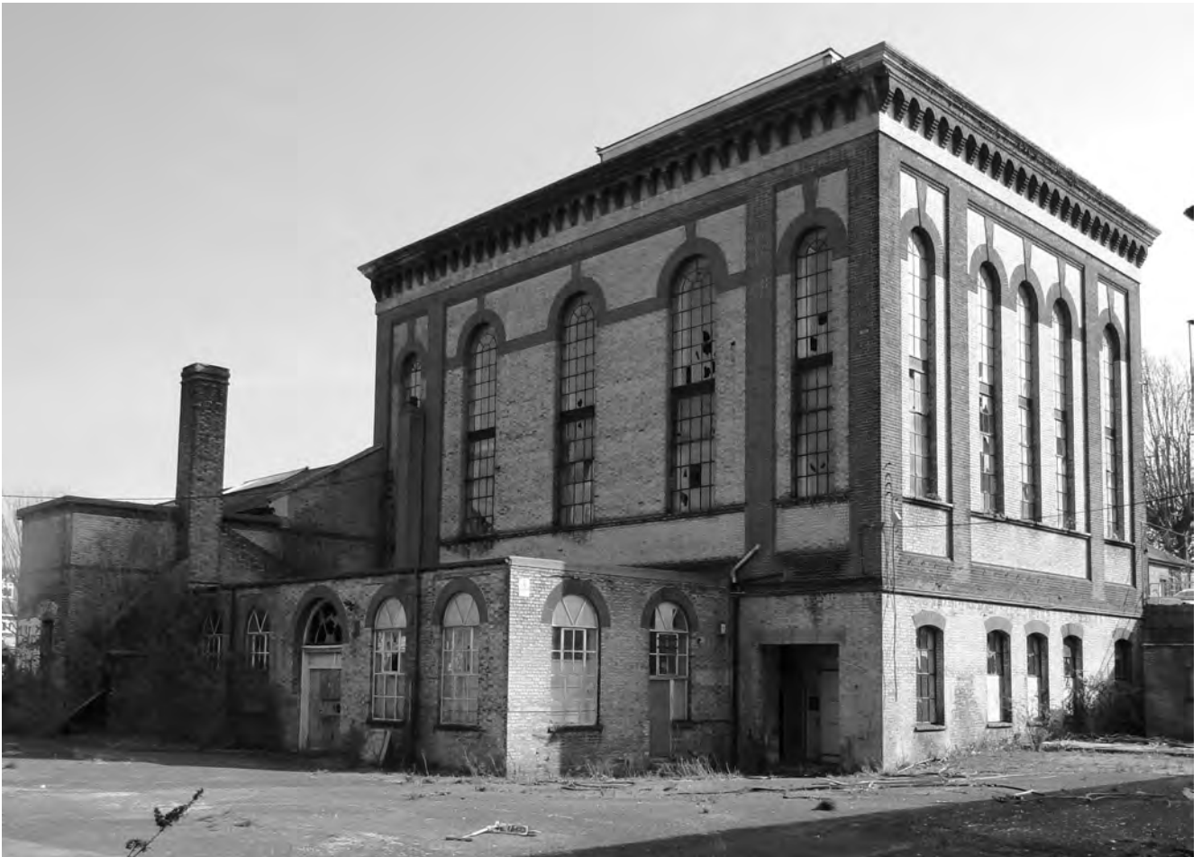
Fig 1. The former pumping station at Bedfordwell
