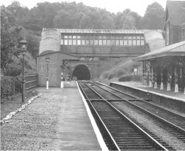
Fig 16. The footbridge at West Hoathly looking towards Horsted Keynes. These footbridges linked into the ends of the canopies so that the transfer from one platform to the next was made in the dry. The canopy of the down platform waiting shelter has been shortened. Although Bluebell Railway trains now pass through here again, there is no trace of the station which was demolished in 1967. (Author's collection)
