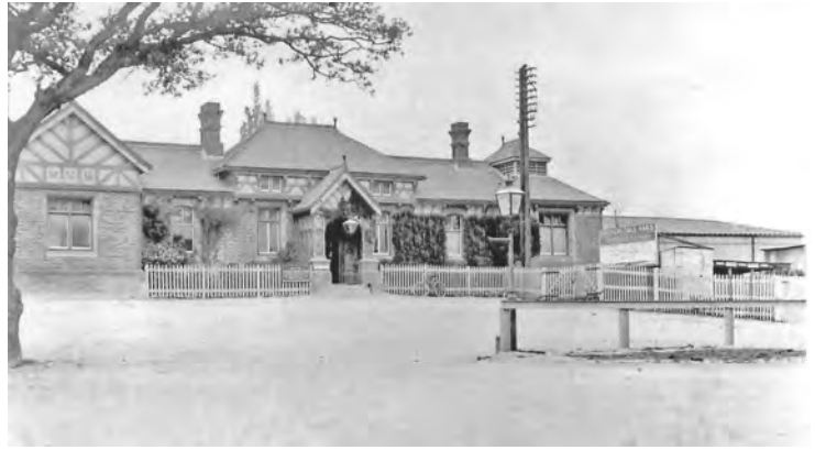
Fig 4. The single storey downside buildings at Hassocks in pre-grouping days. These also featured a transept and again the timbering differs from the later Myres stations. Note the lantern to ventilate the gents' lavatories. (Author's collection)
