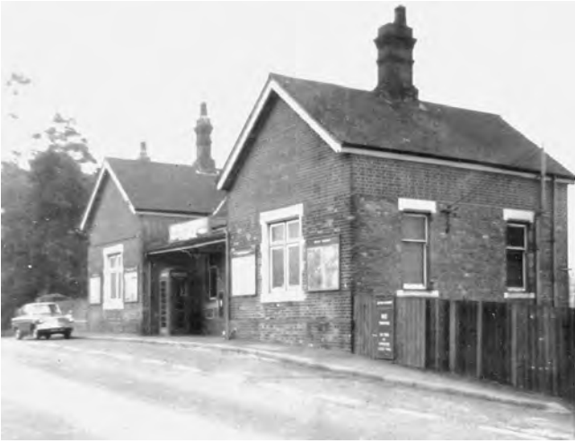
Fig 20. The frontage of Eridge, on the Uckfield Line, seen here in 1968. The buildings are on a bridge above the tracks and incorporate a few Myres features such as those mullioned windows and also the booking office doors which, in this view, are out of sight below the canopy. (Author)
