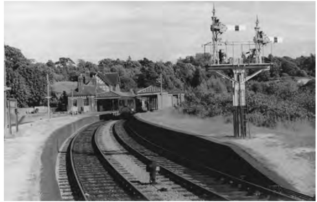
Fig 14. Midhurst (Type 'B') looking towards Selham in BR days, with a push-pull train in the down platform bound for Petersfield. The down platform waiting shelter has an unusually long canopy which, as with all Myres stations, matches that on the main buildings. Note that the station house still sports its mock timbering on this side. Everything here was flattened in 1967 to make way for the Holmbush estate. (T Wright)
