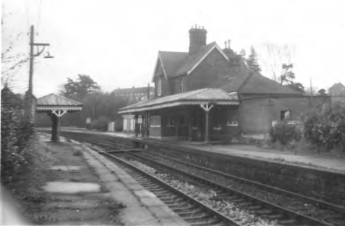
Fig 5. Horam 9 , on the Cuckoo Line, illustrating of the most common layout of a Myres station – which I classify as Type 'A'. Note the commodious hip-ended, zinc-clad canopies and the matching timber waiting shelter on the down platform. Here the mock-timbering has been fully covered with hanging tiles to combat damp penetration. Sadly Horam has long since been demolished but the 'Cuckoo Trail' along the track bed passes its site. (Author)
