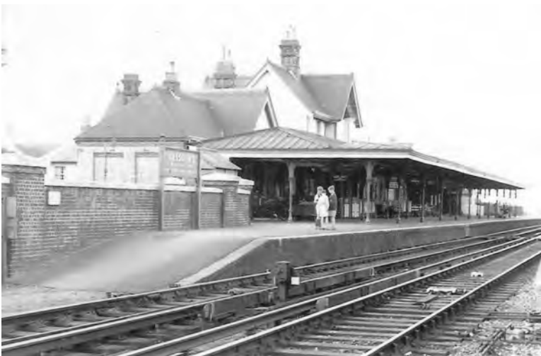
Fig 3. The up platform and main buildings of Hassocks, shewing the canopy-and-a-half. The valances originally matched those of the Cuckoo and Chichester-Midhurst lines but have been reduced in depth, undoubtedly for gauging reasons as those on the down side were not so mutilated. Note that the mock timbering has disappeared from the upper storey. The running-in board exhorts passengers to alight here for Hurstpierpoint College. (Author's collection)
