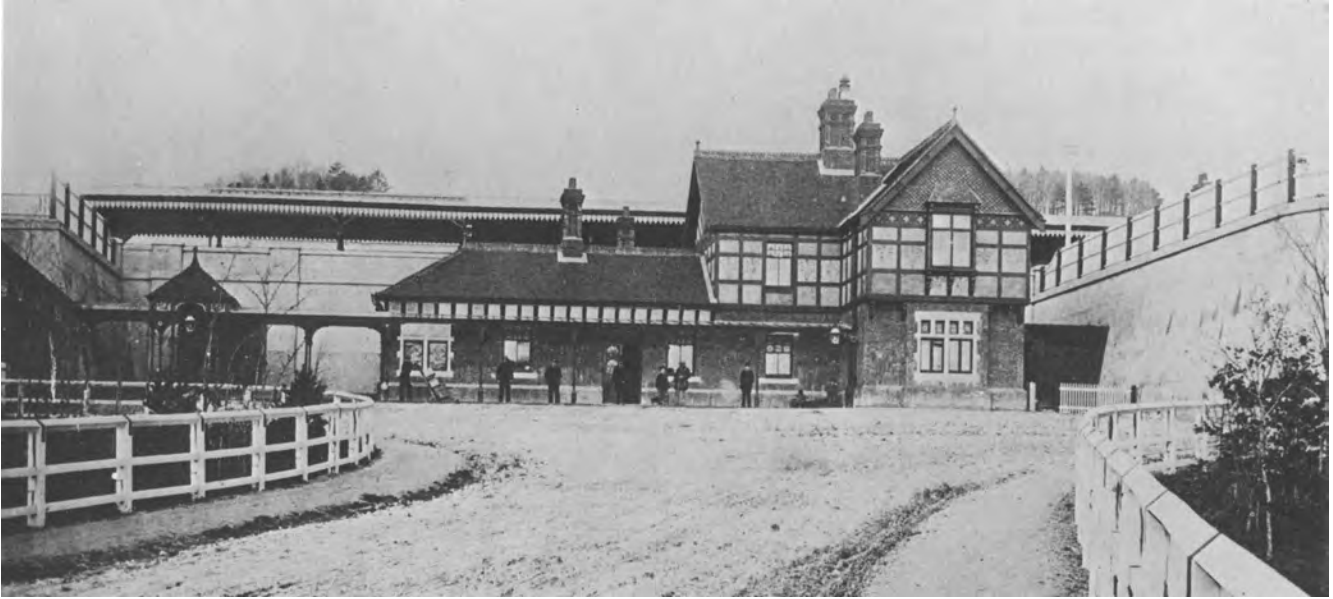
Fig 9. The frontage of Singleton taken from an album of photographs produced in 1881 for Frederick Banister, the LB&SCR Chief Engineer. Behind the main station building can be seen the substantial mass concrete retaining wall with the platform canopies beyond. The isolated building to the left, linked by a veranda, is the vast gentlemen's lavatory. (WSRO)
