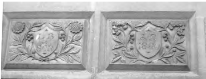
Fig 15.(Left) Cartouches over the ladies' lavatory window at Midhurst displaying the company ownership and the year of construction. These stone mullioned lavatory windows were a standard Myres detail, but on Cuckoo line stations the panels were left blank whilst on the Bluebell line an LB&SCR monogram and the date - 1882- were displayed in cursive characters. (Right) on demolition of Midhurst the cartouches were set into a new wall in the housing estate and survive today, albeit damaged, as the only reminder of the once fine station that occupied the site. (Author)
