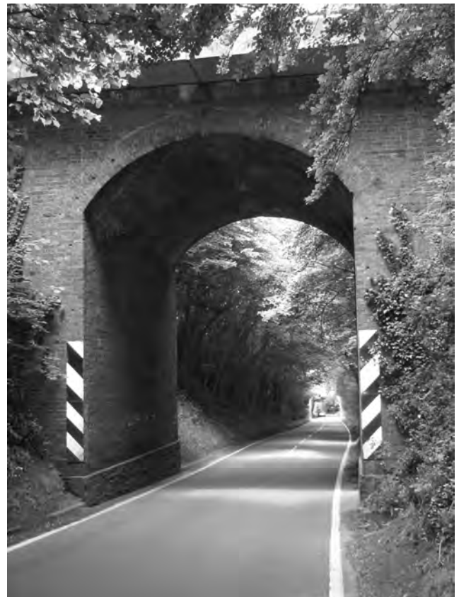
Fig 11. Cripp's Corner flyover
