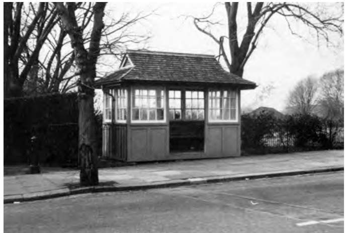
Fig 5. Type 2 shelter opposite Port Hall Road
