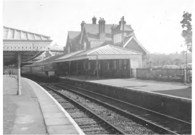
Fig 11. East Grinstead low level seen in April 1968 with '3D' DEMU No 1308 which has just arrived at the low level on a working from Victoria. Behind the train can be seen the canopies of the high-level platforms serving the Three Bridges to Tunbridge Wells line. Note the lantern roof over the refreshment room. The elaborate valances only featured on this line and were soon reduced in depth, probably for gauging reasons, on all stations, but at East Grinstead they survived on the ends of the low-level canopies. (Author)
