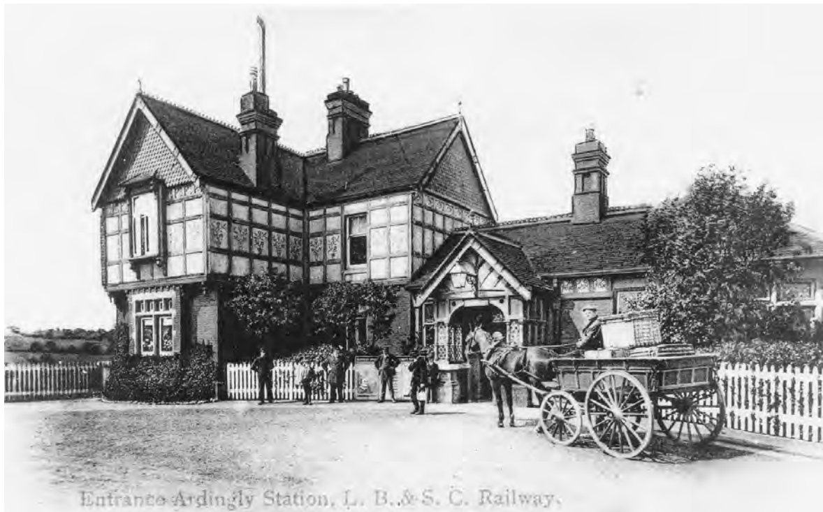
Fig 1. The frontage of Ardingly by T H Myres seen in pre-grouping days. This shews a Myres station in all its as-built glory with the characteristic mock-timbering and pargetting of the upper storey, oriel window and porch with stained glass windows. This building is still with us but the upper storey has lost its timbering and the chimneys have recently gone. (Author's collection)
