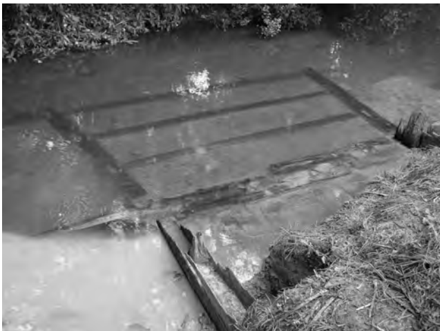
Fig 2. The frame and boards exposed to the first uprights
