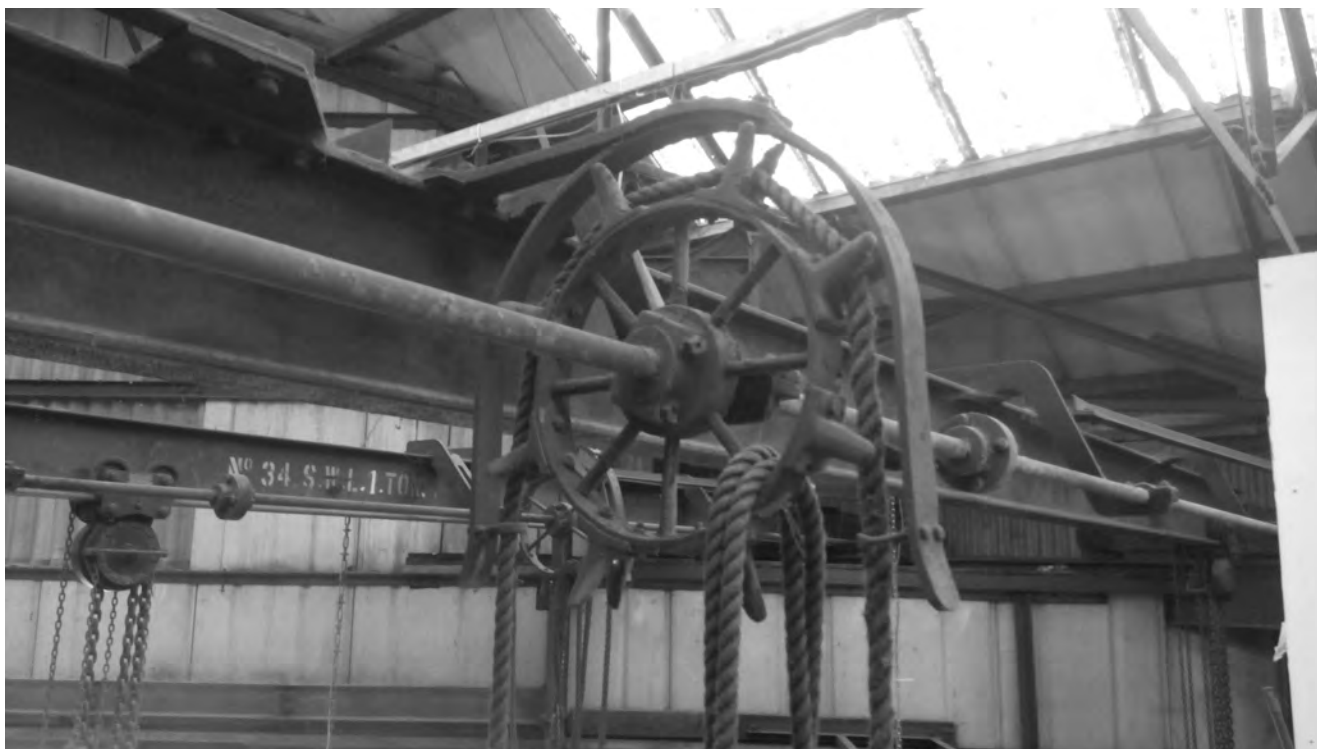
Fig. 9 The surviving chain and pulley hoist mechanism in Shed 6
