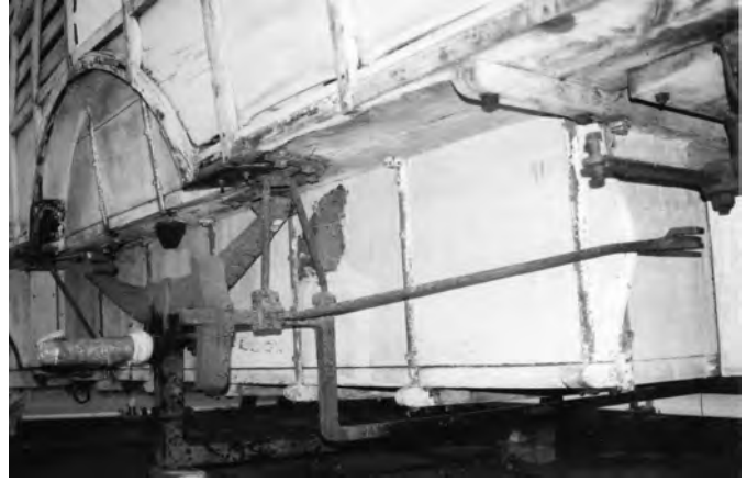
Fig. 8 Details of well bottom and brake gear as found
