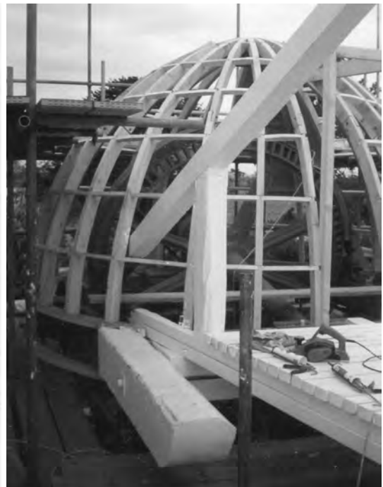
Fig. 15 Barnham, restored caps with new ribs, 1999 (Photo by P. Hicks)
