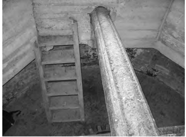
Fig. 19 Selsey Mill, internal ladder (next to tail of windshaft) which travelled round with cap (Photo by P. Hicks)
