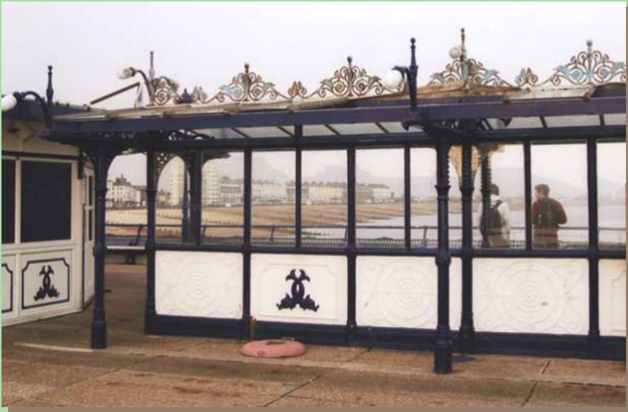
Windscreen on Eastbourne Pier, with iron work made by John Every at the Phoenix Iron Works, Lewes
