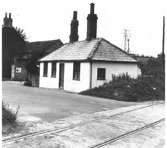
Fig. 10 Southeram tollhouse, July 1937 (Frank Gregory)
