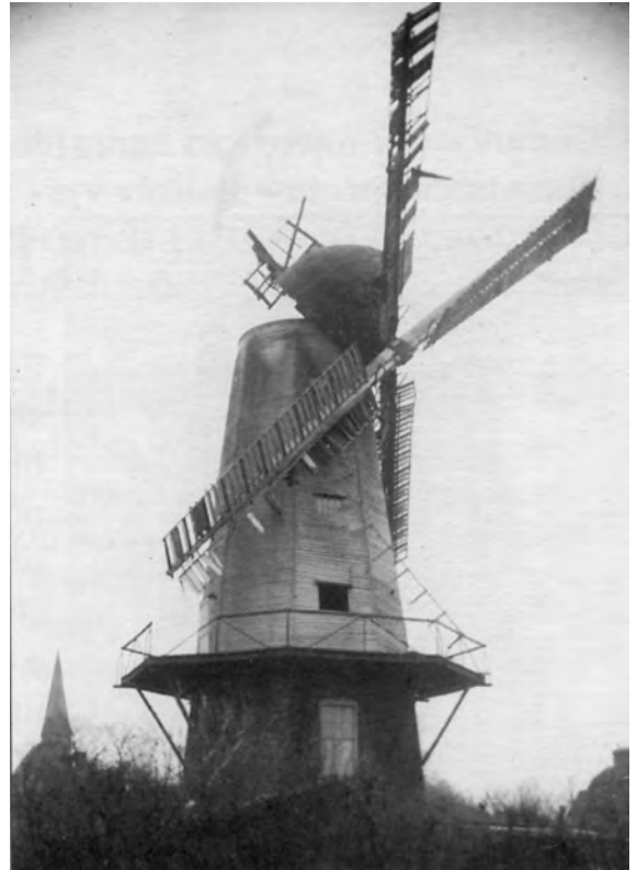
Fig. 12 Wisborough Green Mill tail-winded (Image courtesy of Eileen Finch)
