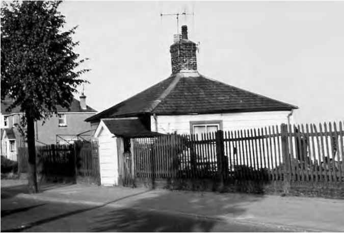
Fig. 4 Crumble Bridge tollhouse just before demolition in early 1964
