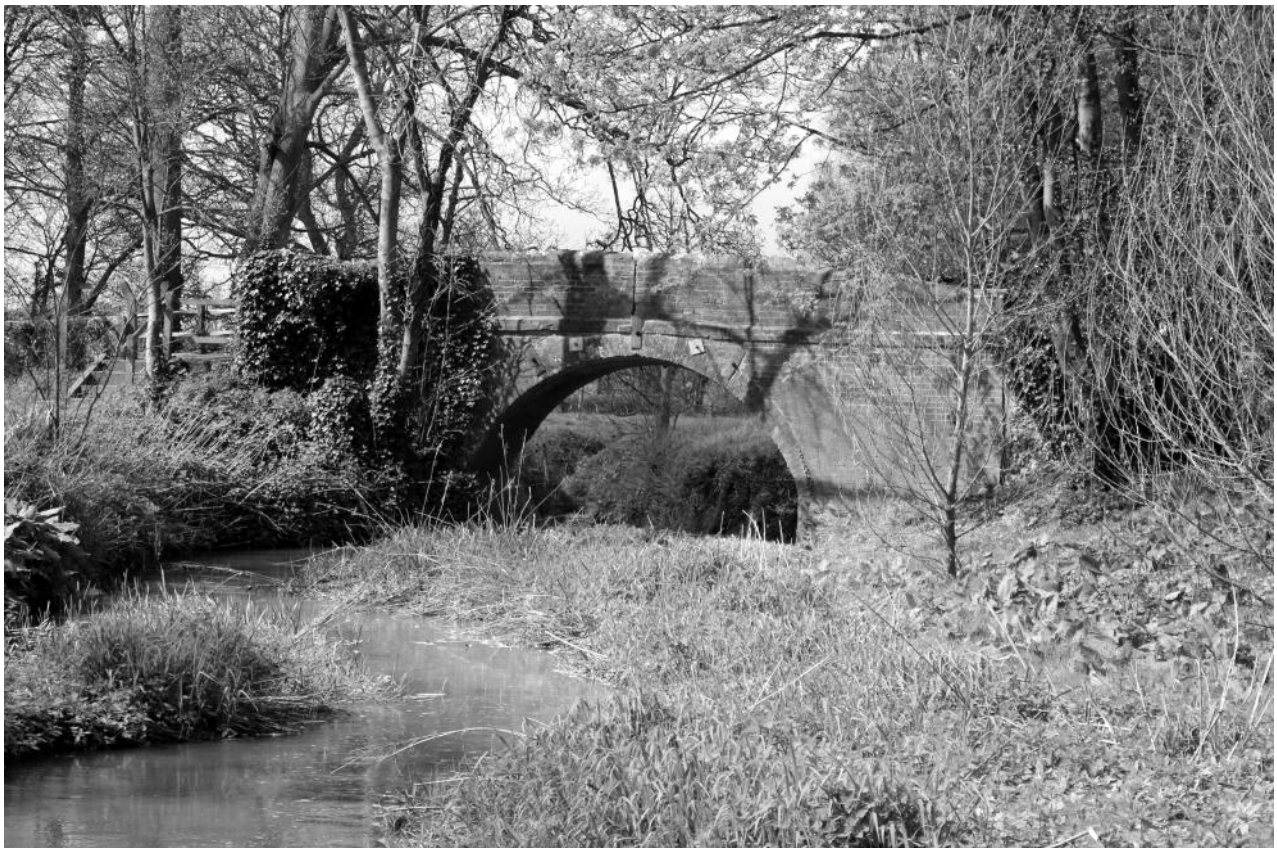
Fig. 4 Pikes Bridge photographed in April 2014 (Nick Kelly)
