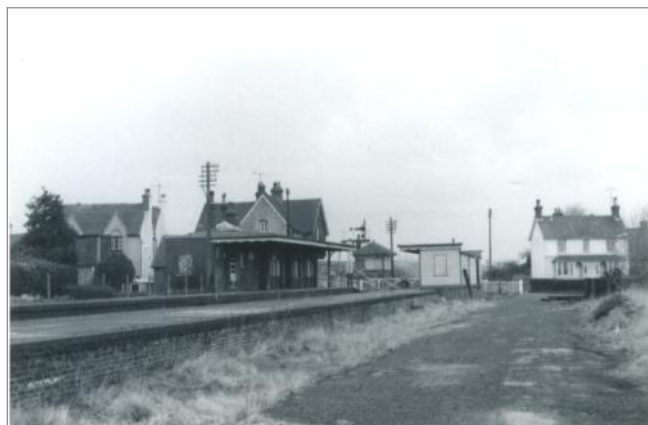
Fig 13. Barcombe Mills in 1970 after closure and awaiting track lifting. The buildings and signal box have been boarded up and vegetation is taking over the track, but curiously the signal arm has not been removed. This view shews the downside buildings at the far end of which can be seen the loading bay to the goods shed.
