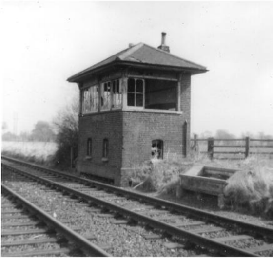
Fig. 10 Culver Junction signal box, which had closed in 1958, seen still standing ten years later but looking somewhat past its prime. Barcombe Mills to Lewes Main Junction was now worked as one long block section. (Author)
