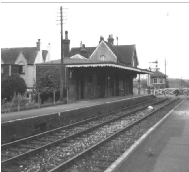
Fig. 6 Barcombe Mills looking north in 1968. Apart from the SR pattern crossing gates and bracket signal little has changed since the view in Fig 1 was taken. The white building behind the station is The Anglers' Rest public house. (Author)
