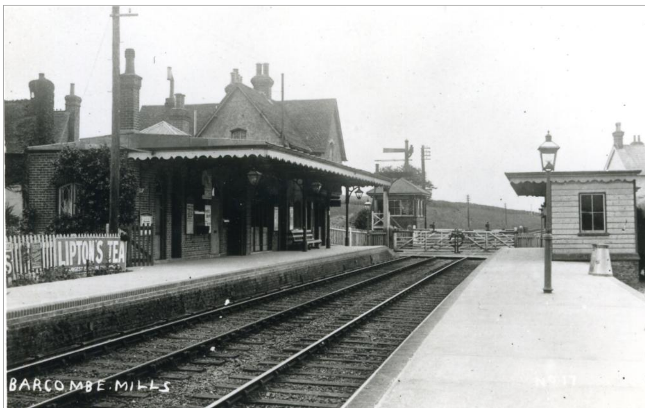
Fig. 1 A postcard view of Barcombe Mills station when in pure LBSC condition. The view is looking towards Isfield with the signal box beyond the level crossing. Being remote, the station was lit by oil rather than gas right up until closure in 1969. Note the milk churn on the down platform. (Author's collection)
