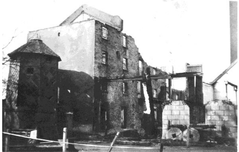
Fig. 13 View from the north-east showing the former corn-drying kiln, remains of the warehouse and engine house.
