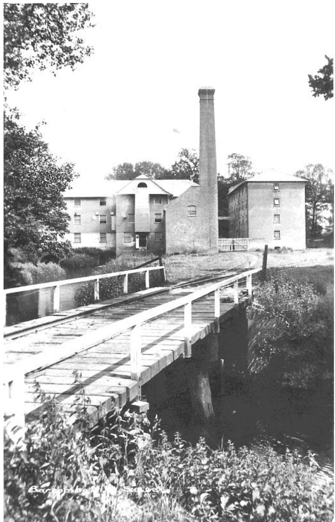
Fig. 4. Rear view of the mill with the railway siding crossing the bridge over the mill race, the former corn mill to the left, and the engine house and warehouse to the right.
