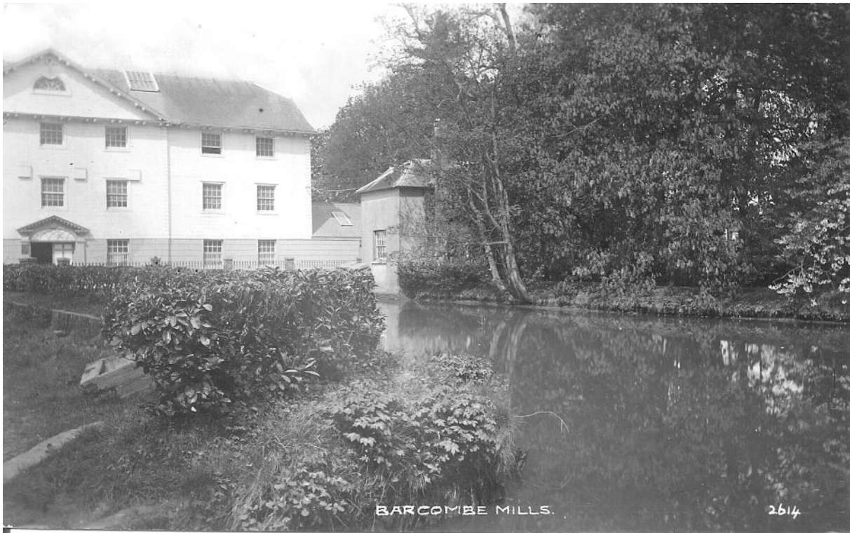
Fig. 2 East side and front of the former corn mill, showing the Carpenters' Shop, Wharf Cottage and the mill pond
