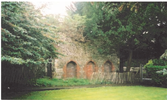
Fig. 2 North side of the pump house
