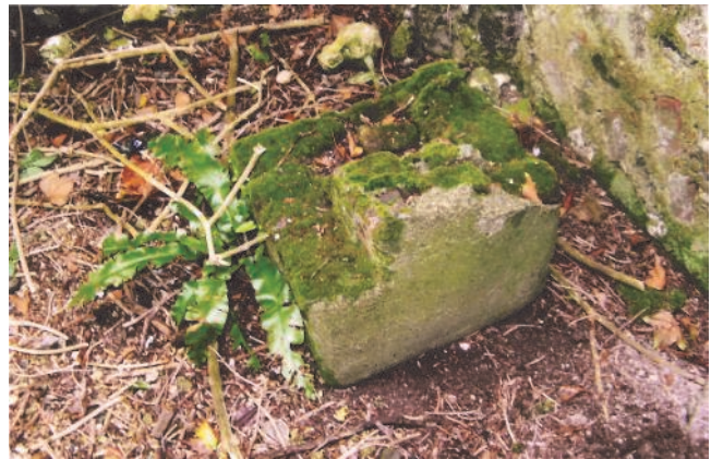
Fig. 8 Fragment of brick work on the ground
