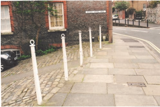
Fig. 7 Top chain rings and two sleeved repairs (author)
