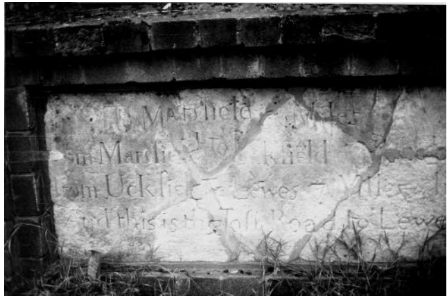
Fig. 6 Sandstone panel listing mileages to Lewes originally in the wall of Wych Cross tollhouse
