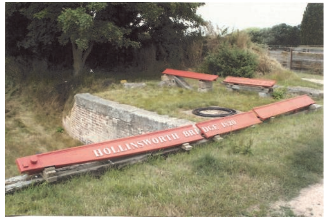
Fig.3 Parts of Hollinsworth bridge at the Stewart Bridge site on Barnham Court Farm (author)
