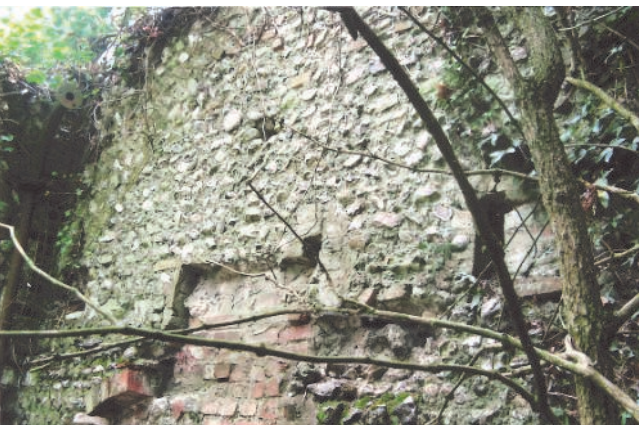
Fig. 11 Oblong recesses in the south wall
