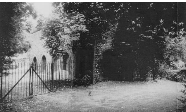
Fig. 5 Well house with later raised walls and eastern extension (K. Gravett, June 1963). By permission of English Heritage NMR.
