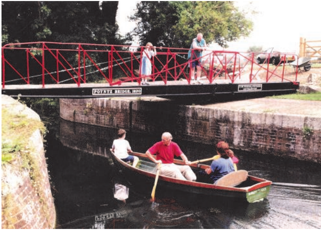
Fig.2 Poyntz Bridge in closed position
