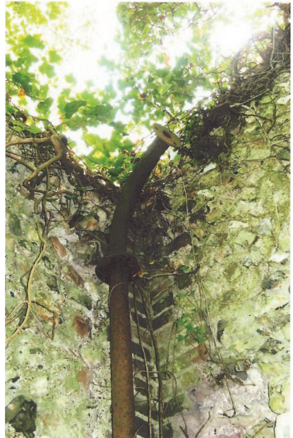
Fig. 12 Water pipe in the south-east corner
