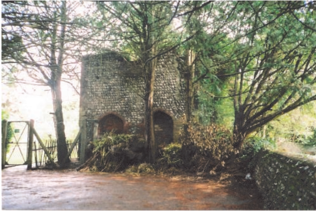
Fig. 1 Preston Manor Pump House (west side)
