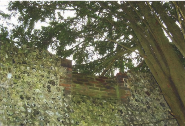
Fig. 10 Blocked window in the west wall
