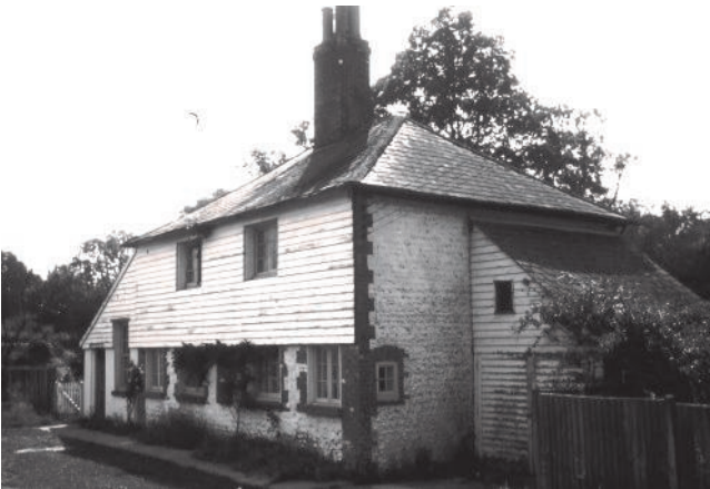
Fig. 11 Hickstead tollhouse c.1975
