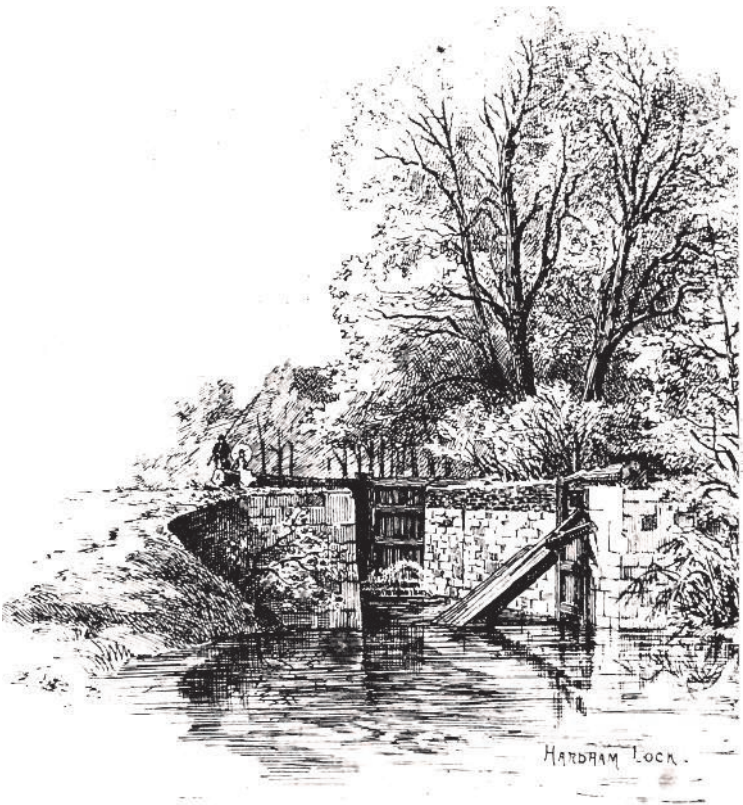
Fig. 11 The entrance to Hardham (Neil's) Lock, 1889
