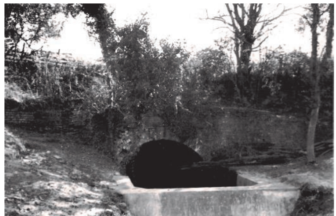
Fig. 8 The North Entrance, 1952. The concrete dam was newly erected on the site of Tunnel Lock.
