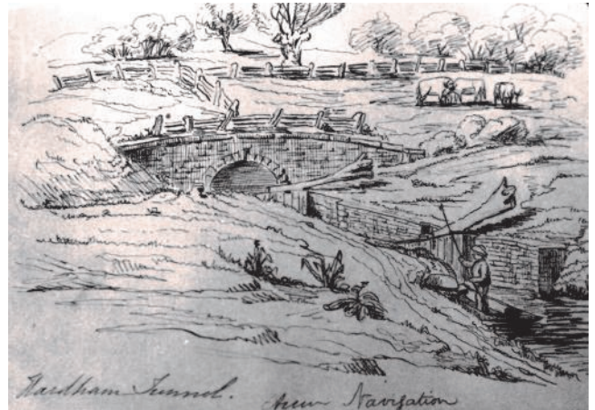
Fig. 6 The North Entrance and Tunnel Lock from a drawing by Thomas Evershed, 1843. Observe the tree trunks used as crude beams for the lock gates.
