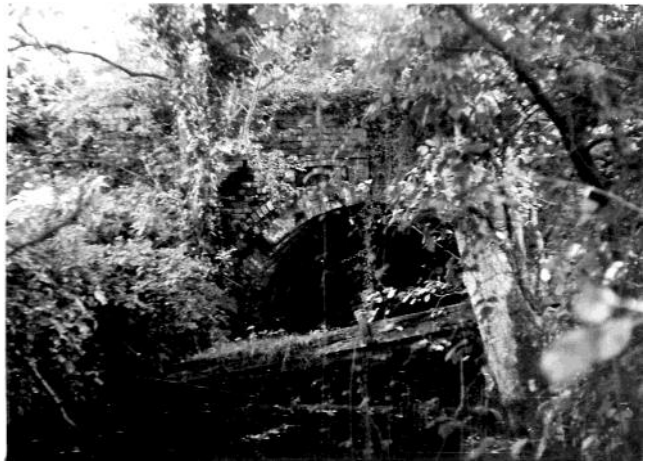
Fig. 7 The remains of the upper gate of Tunnel Lock, 1951
