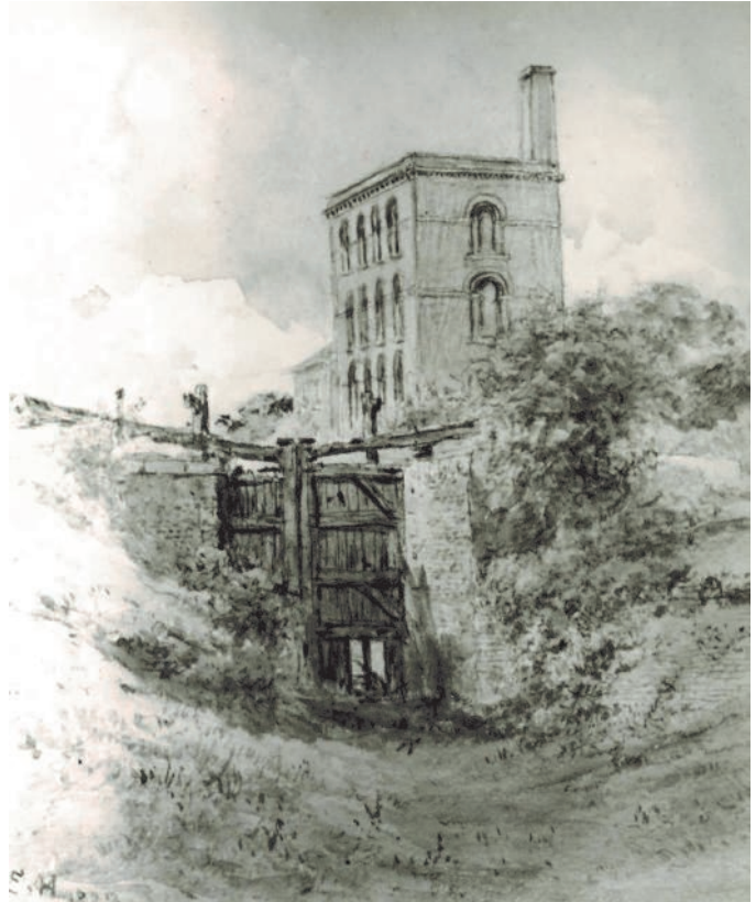
Fig. 1 A painting, dated 1888, of the top (No. 2) lock at Ford, with the pumping station in the background, one of the few images we have of this significant engineering feature of the Portsmouth & Arundel Navigation. At this time the canal had long-been disused; the lack of water and the derelict state of the lock gates will noted. (WSRO)
