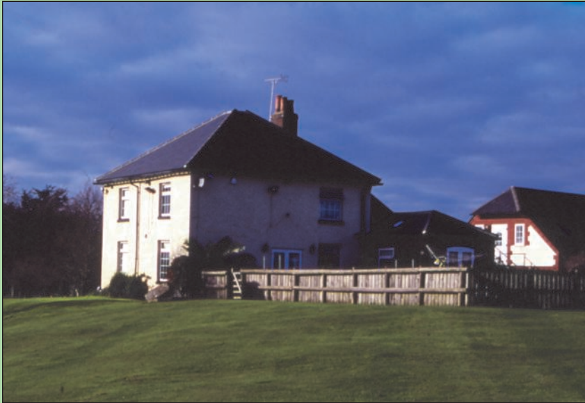
The surviving cottages at Ford built to house the engine and lock-keepers (Alan Green)
