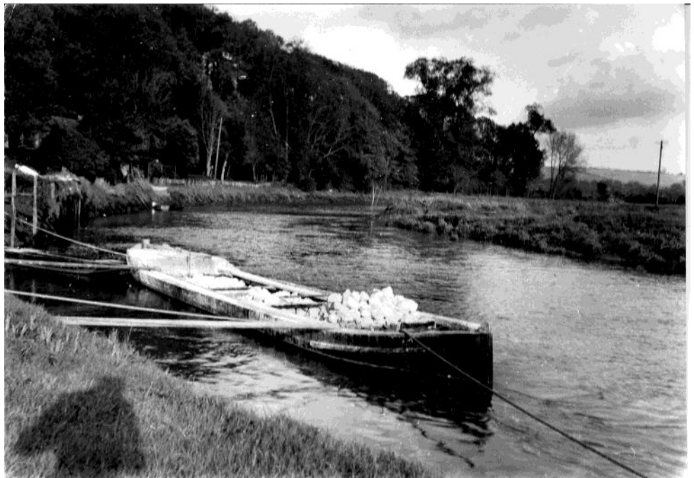
Fig. 18 River Arun Catchment Board barge, 1944. Until the 1950s these barges loaded with chalk blocks were used for bank protection. Similar barge types had regularly used the tunnel loaded with 30 tons or more of chalk for the lime kilns.
