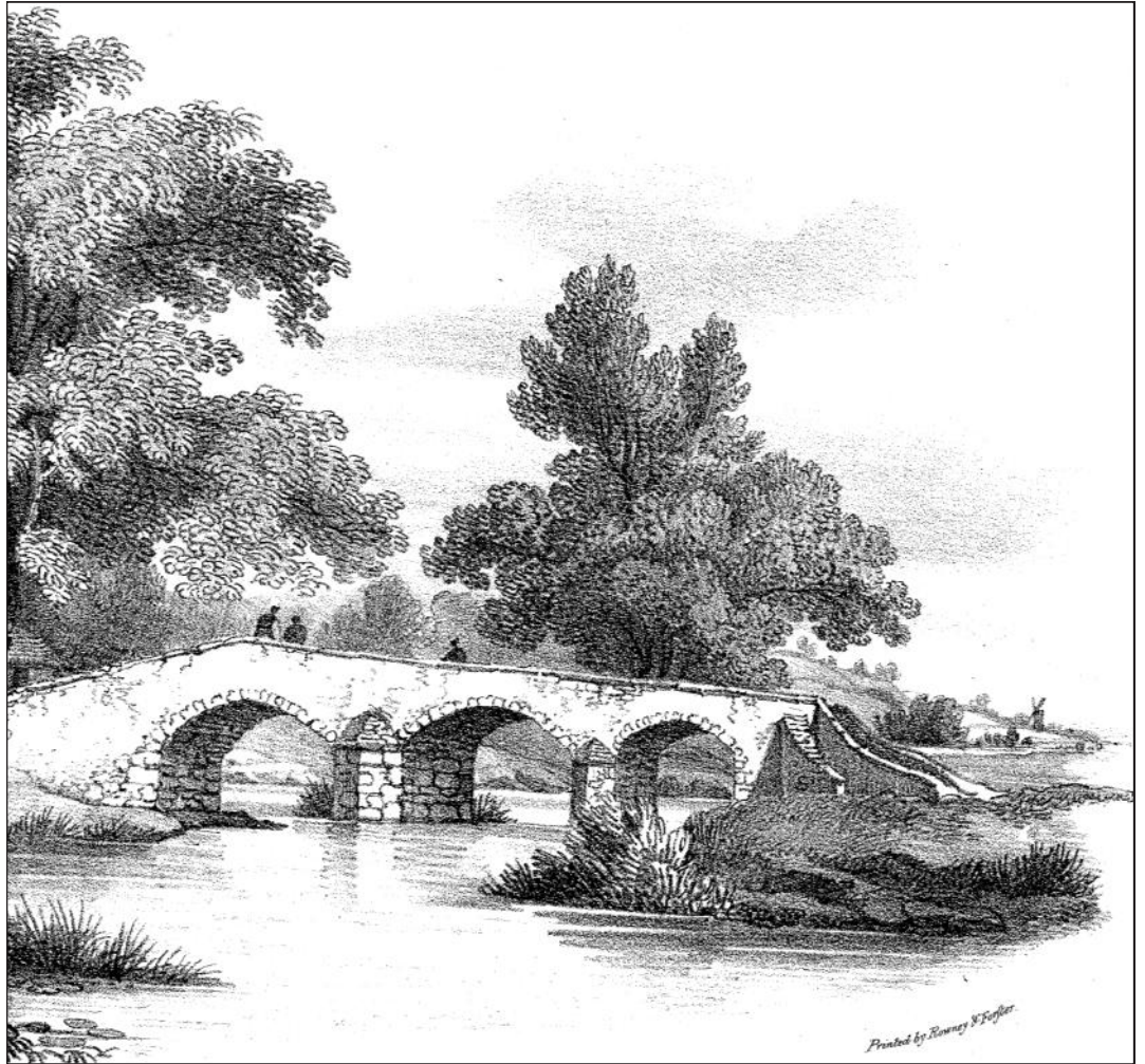
Fig. 13 Clements Bridge, Pulborough, drawn here in 1826, was built in the 1790s. Its ostensible purpose was to provide access for cattle to the water meadows, but its low arches suggest that its main object was to discourage barge traffic from using the toll-free river instead of Hardham Tunnel. Pulborough Church is visible at the left.
