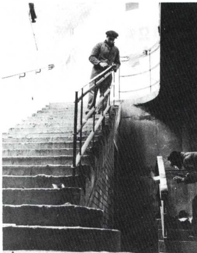
Putting the finishing touches to the guard rail on the steps from the tunnel to the terminal
