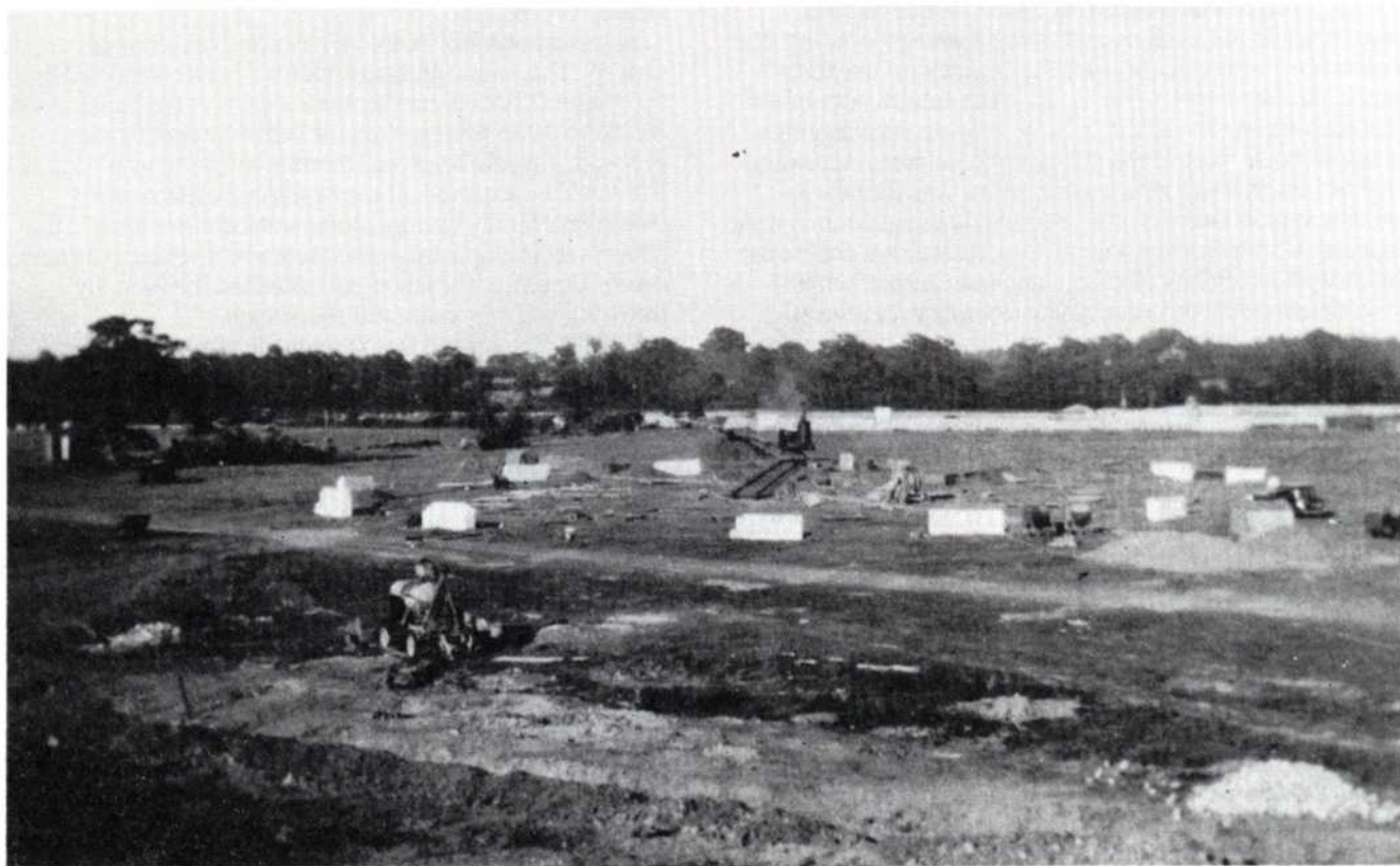
Concreting work in progress. Note the narrow gauge railway (D. Dalton)
