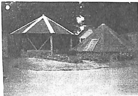
The gin and pump are contained in two separate buildings located 50 yards or so to the north of the Hall. Both buildings are octagonal and similar in plan size with sides about 8 feet long built of bricks laid in Flemish bond to a height of some 2 feet externally. In the case of the gin
